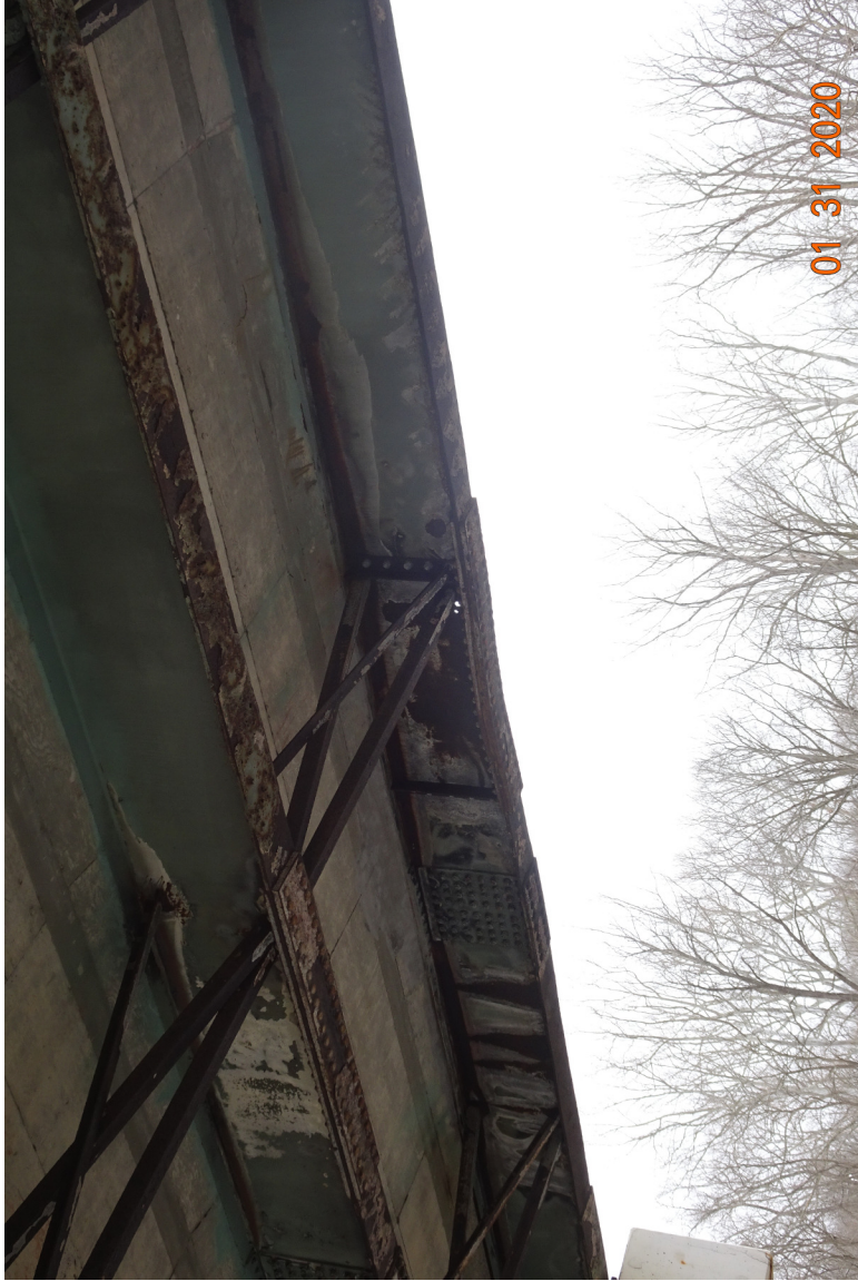
Collision damage to beams 1 and 2 over eastbound US 422
