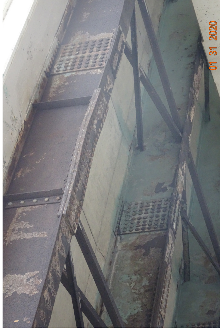
Collision damage to beams 1 and 2 over eastbound US 422
