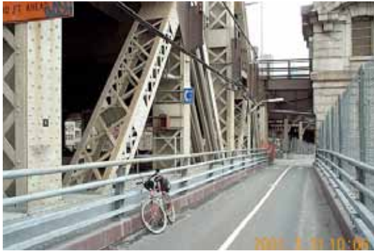
EMERGENCY CALL BOX located on the Queensboro Bridge in New York
