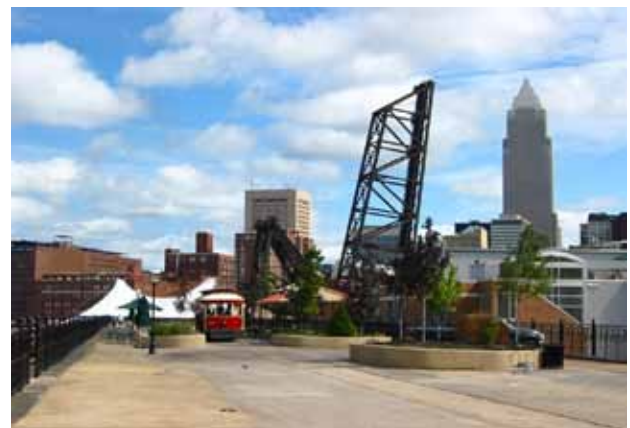
View from the edge of the Superior Viaduct
