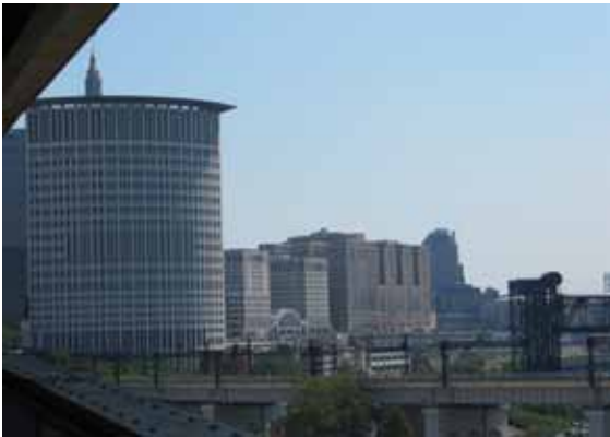
Tower of the former Cleveland Milling Co. adjacent to the bridge, seen from the southern bay, west of the center span.
