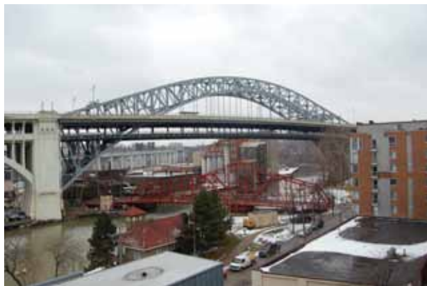
CENTER STREET SWING BRIDGE provides access to the site of the future Canal Basin Park
