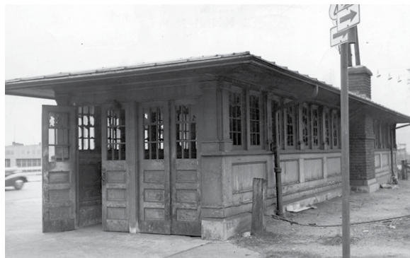
FORMER SHELTER over ramp at W. 25th & Detroit Avenue
