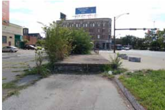
ACCESS RAMP currently sealed at the west end
