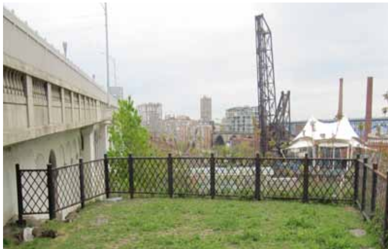
View from bridge platform to Flats
