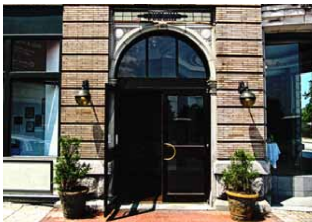
FORMER ENTRY To the streetcar level of the bridge. While the connection still exists, today the entry leads to a restaurant
