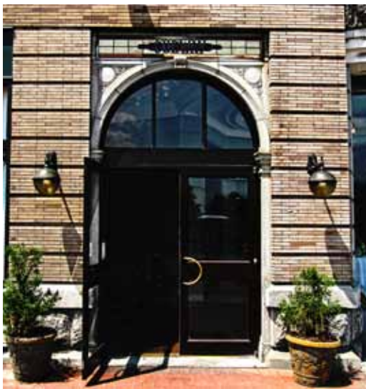
FORMER ENTRY leading from the “Forest City Savings and Trust Building”
