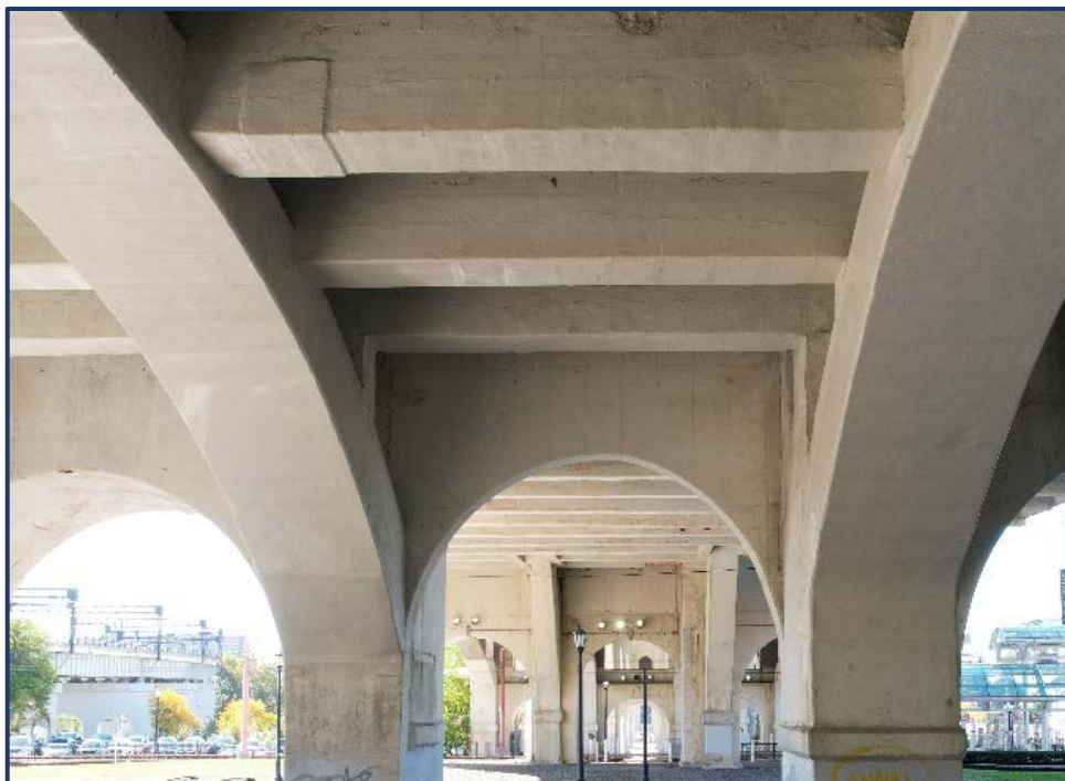
Photo 155-6 – Span 13, FRP on Underside of Lower Deck Floorbeams
