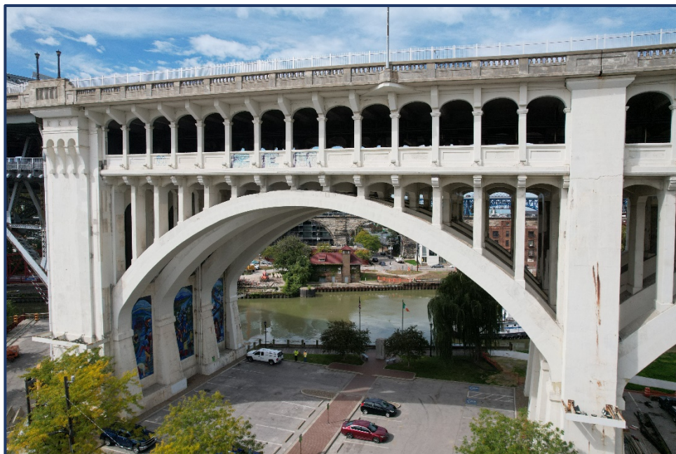
Photo 144-1 – Span 5 Reinforced Concrete Arches
