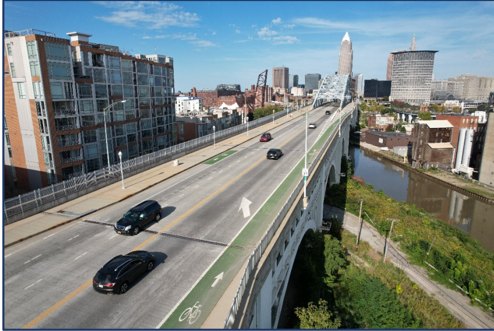
West End of Bridge, Looking East
