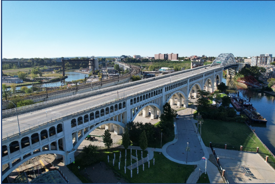
North Elevation of Bridge, Looking Southwest
