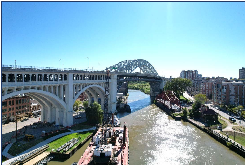
Photo CH-2 – Downstream Channel, Looking South
