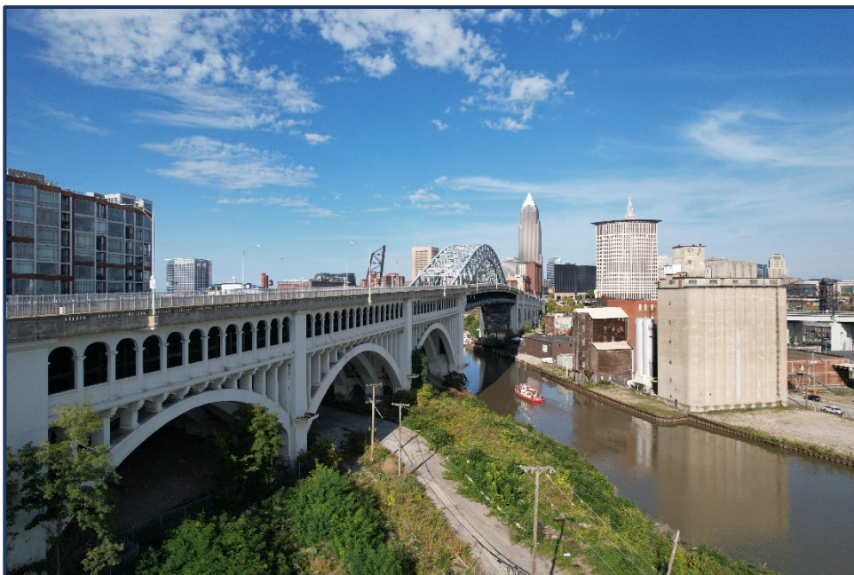
South Elevation of Bridge, Looking Northeast
