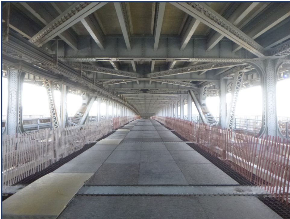
View of Span 4 Maintenance Deck, Looking West
