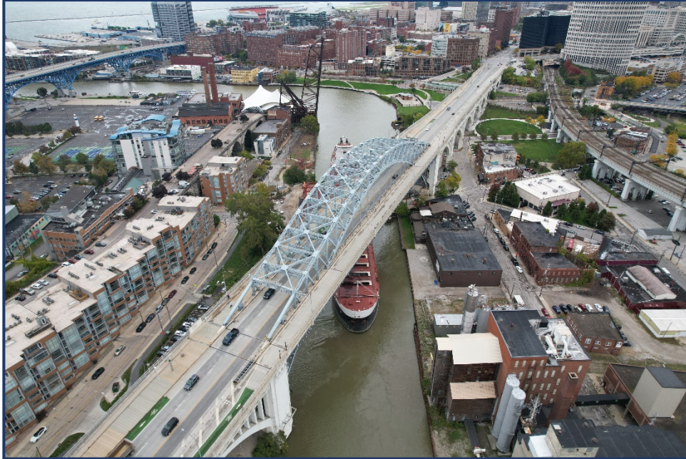
Main Truss Span (Span 4), Looking Southwest
