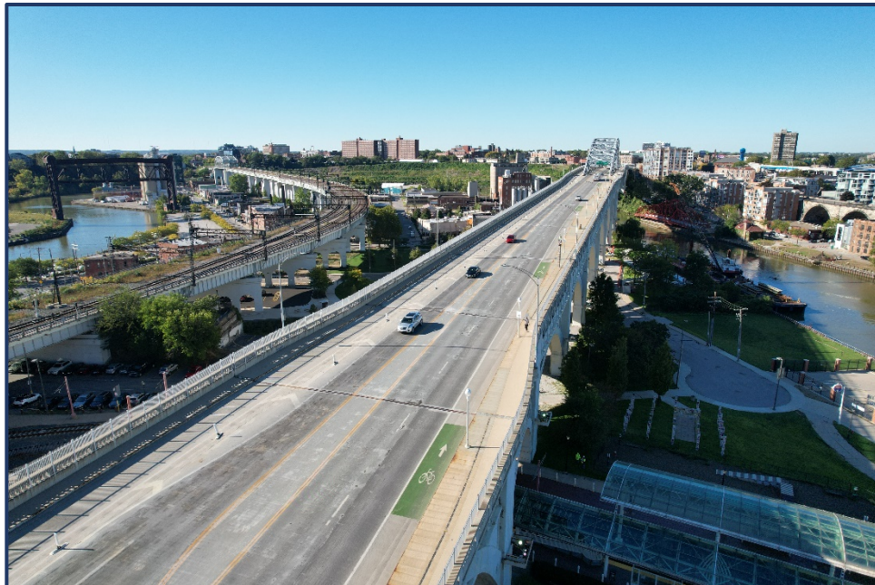
East End of Bridge, Looking West
