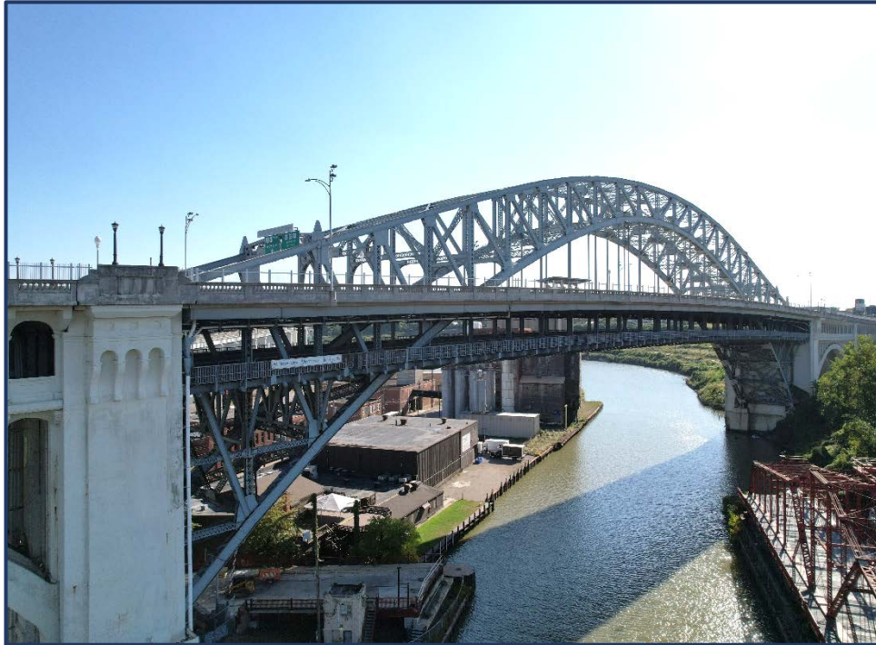
Photo 120-1 – Span 4, North Elevation of Truss
