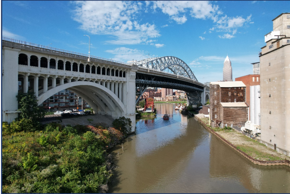
Photo CH-1 – Upstream Channel, Looking North
