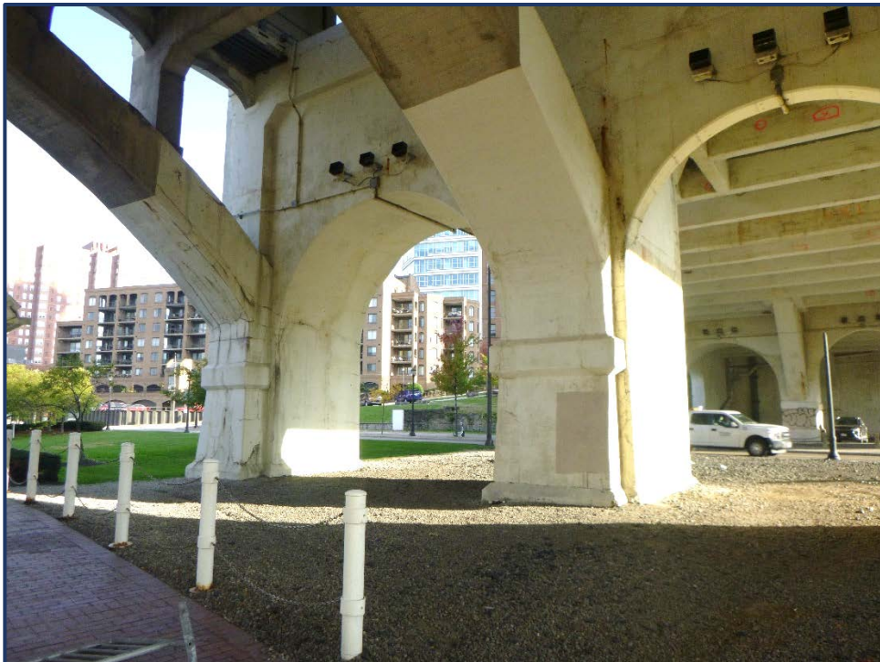
Photo 205-2 – Pier 11, West Face
