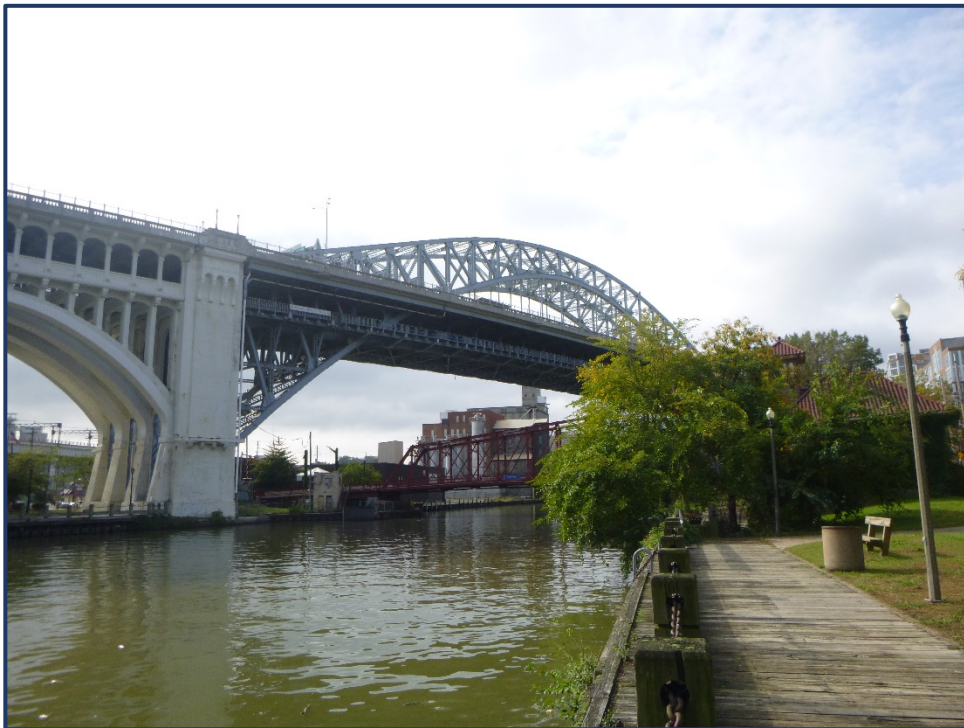
North Elevation of Span 4, Looking South
