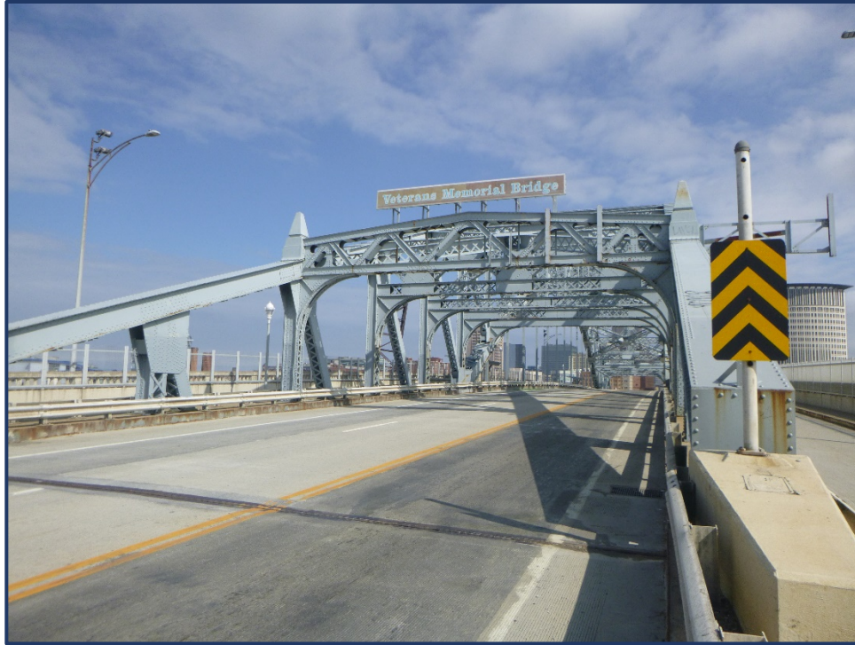
Main Truss Span (Span 4), Looking West
