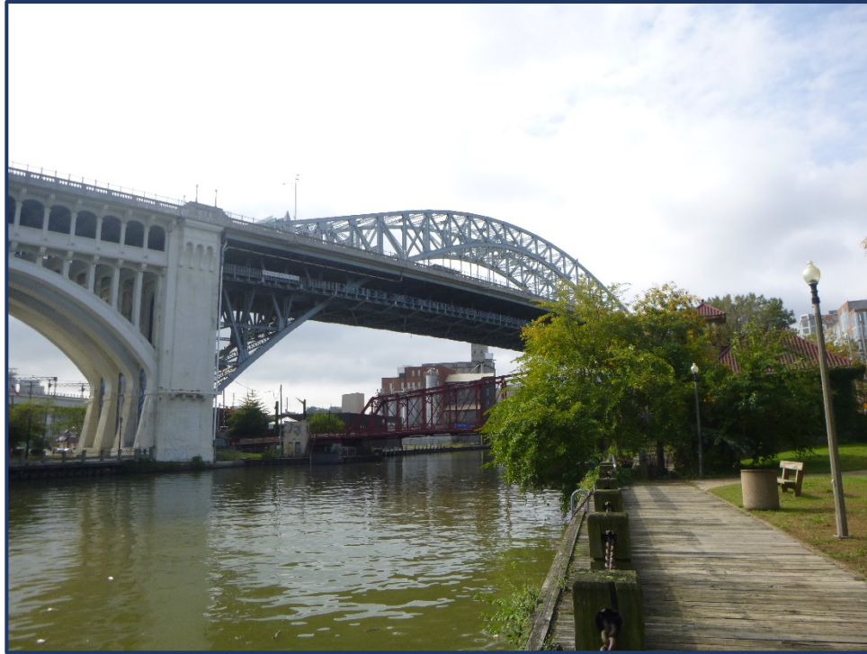
Photo CH-1 – Downstream Channel, Looking South
