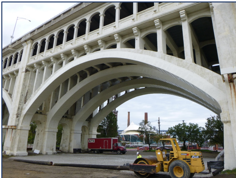
Photo 144-1 – Span 9 Reinforced Concrete Arches
