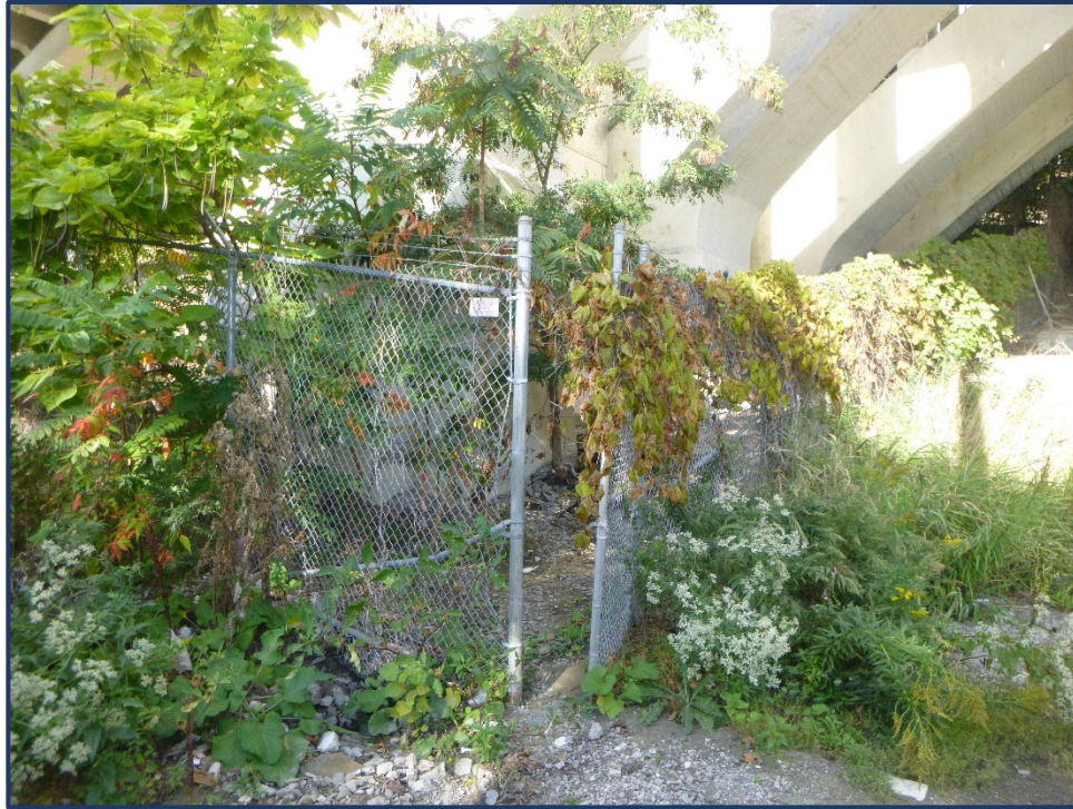
Photo APR-3 – Open Fence at Southeast Corner of Pier 1
