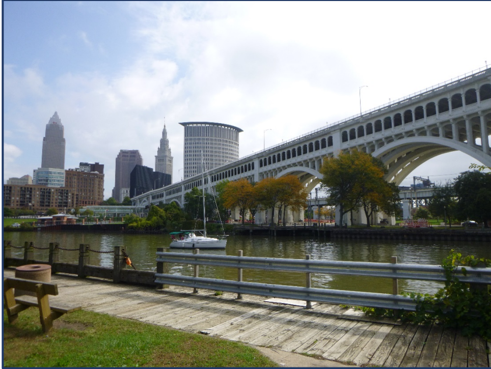
North Elevation of Bridge, Looking Southeast
