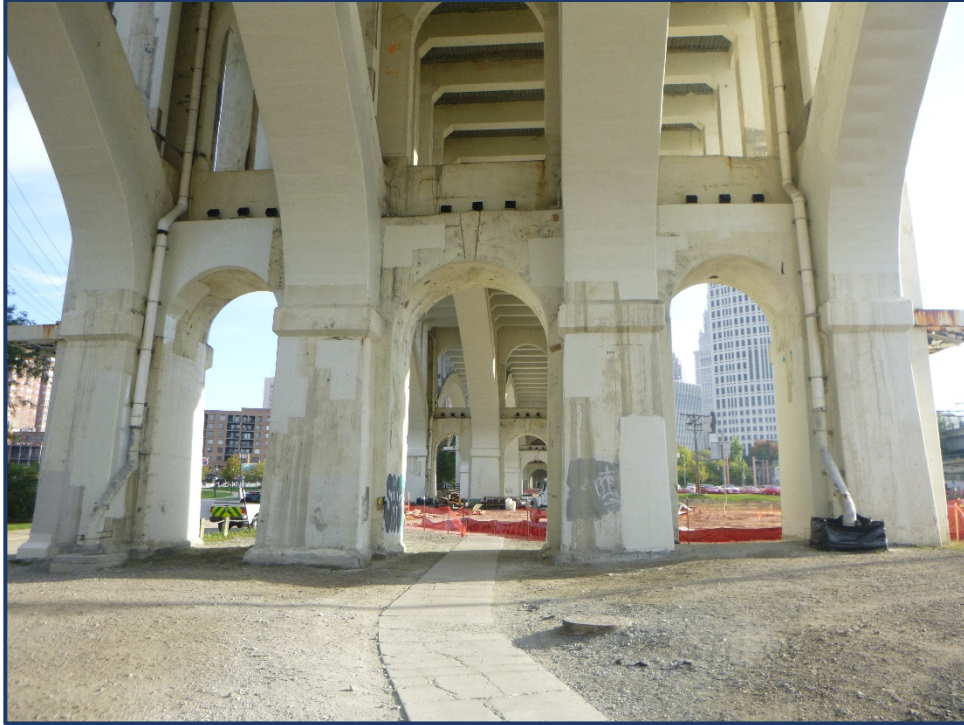
Photo 205-1 – Pier 7, West Face
