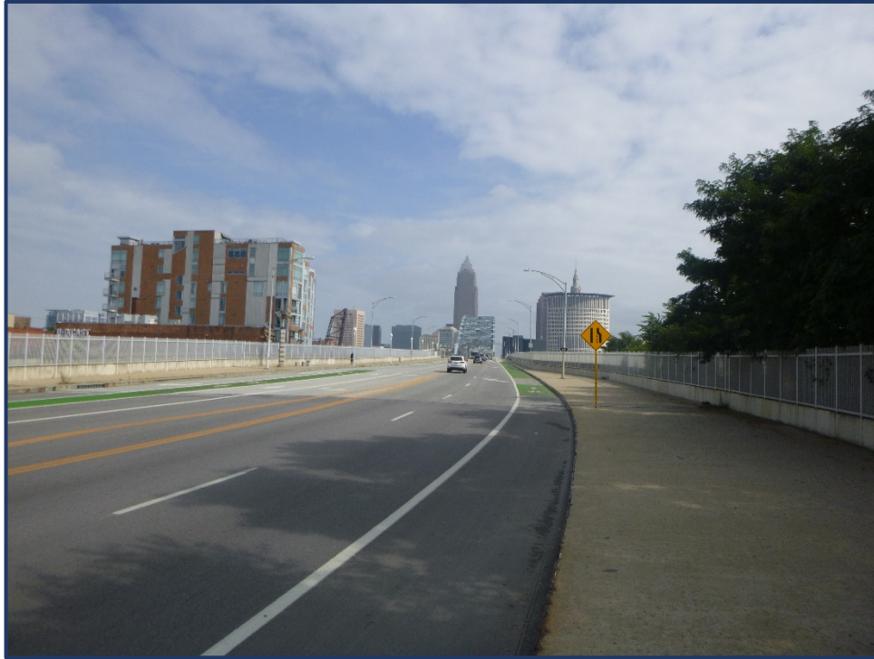
West End of Bridge, Looking East
