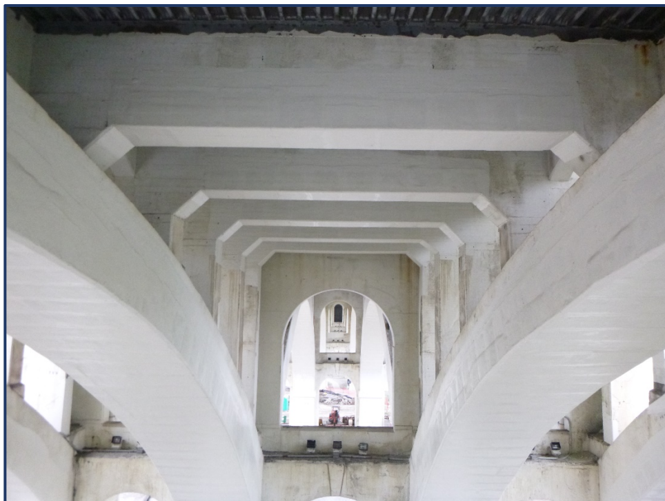
Photo 155-5 – Span 10, FRP on Underside of Lower Deck Floorbeams
