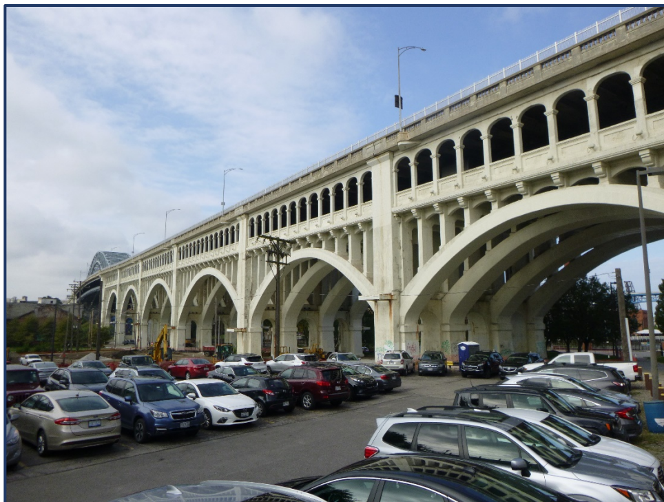
South Elevation of Bridge, Looking Northwest
