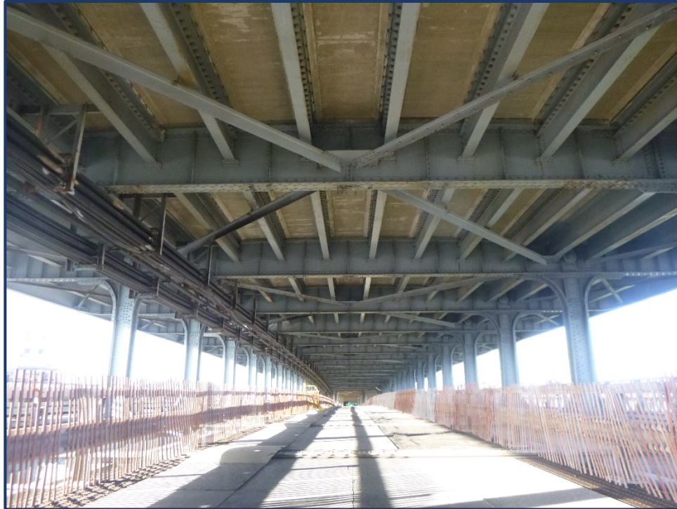
Photo 12-5 – View of Deck from Maintenance Deck, Span 4, Center Section
