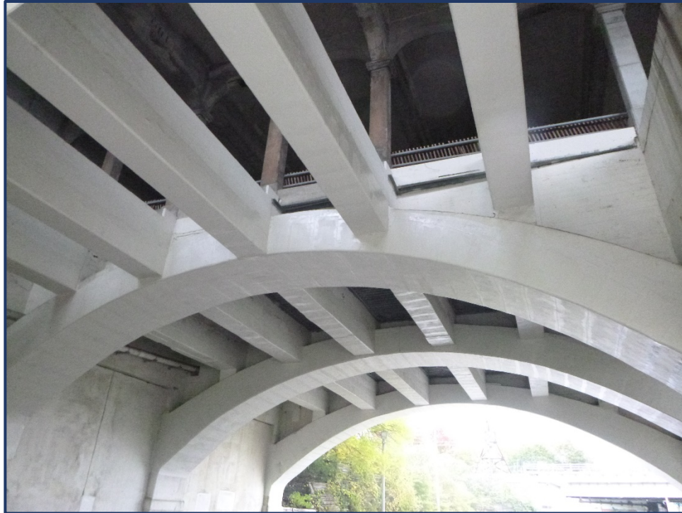
Photo 144-2 – Span 13, FRP on Underside of Concrete Arches
