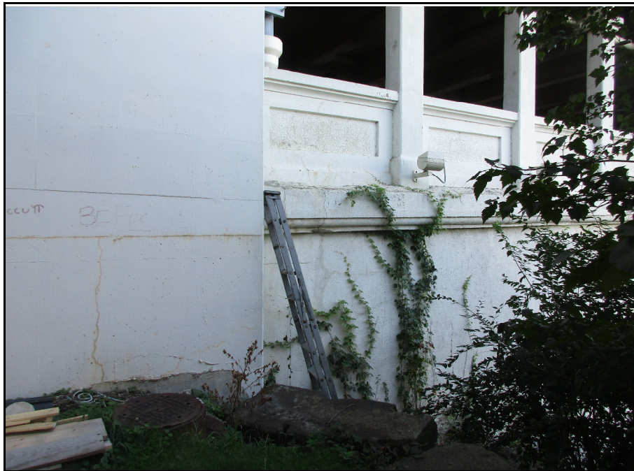
Photo 9 – Ladder Used by Vandals to Access Lower Deck, Span 13 at East Abutment.
