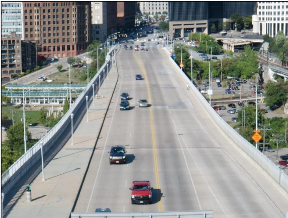
Photo 2– East Approach Spans Deck, Looking East.
