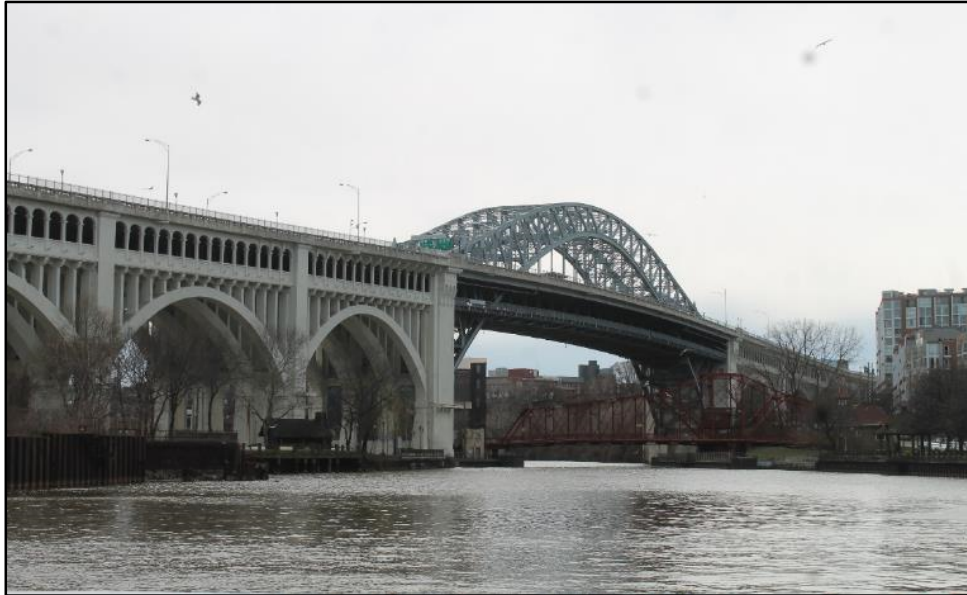
Photo 1– North Elevation, Spans 4 through 6.
