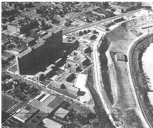
Figure 4: Graded Site with Realigned Franklin Avenue
