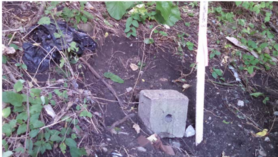
Figure 16: Horizontal 2" Diameter Drain Pipes Installed in 1966
