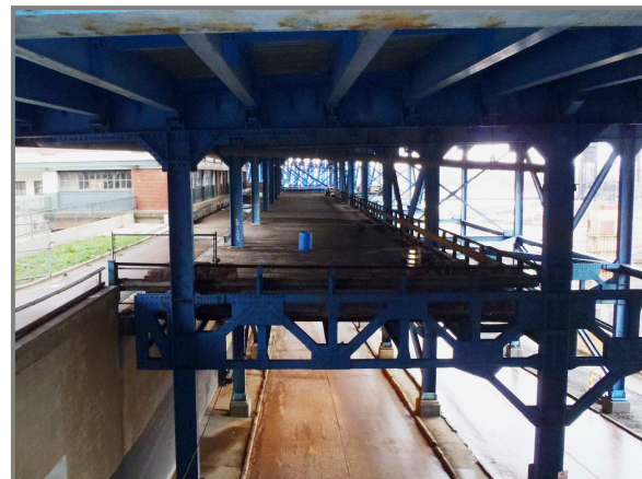
Photo 12 – Lower level deck in the East Approach – Forward Section (looking west)
