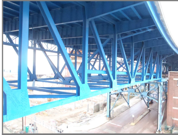
Photo 10 – South elevation of Span 11 (looking east)
