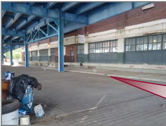
Photo 18 – Looking south from lower deck at apartment building and lower deck.
