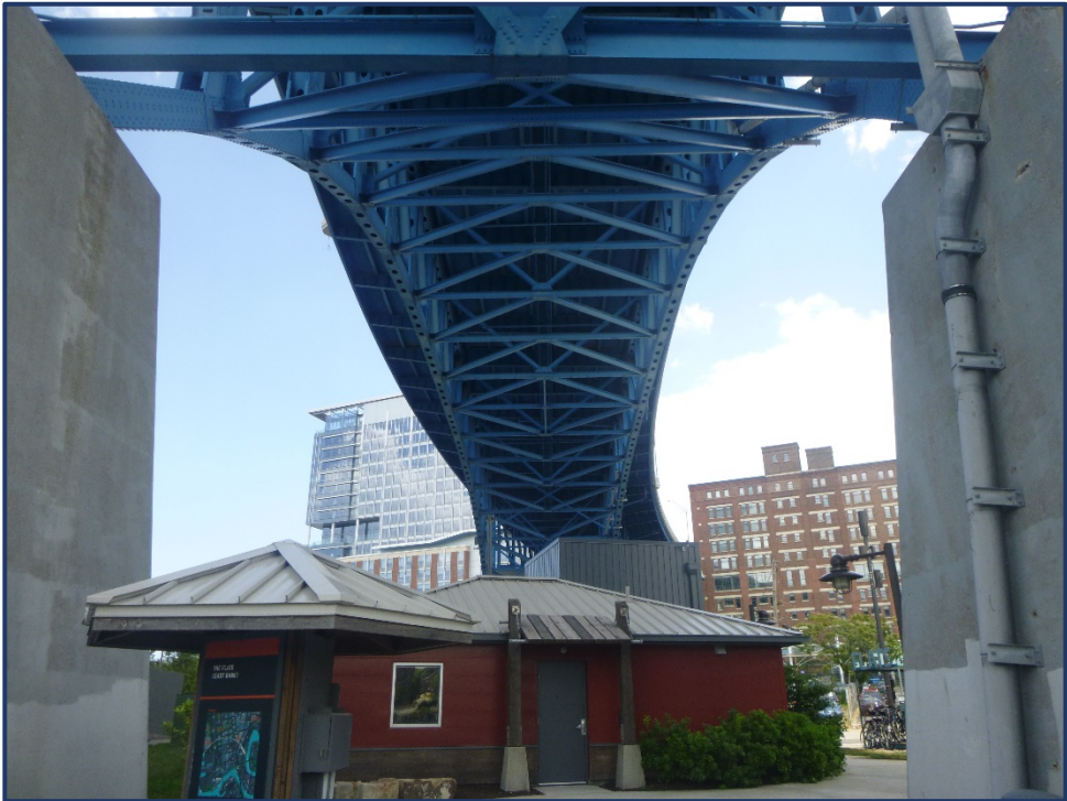
Unit II Span 10 Typical Superstructure Looking West
