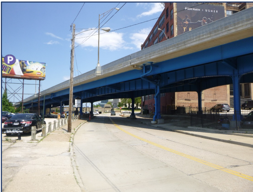
Unit IV North Elevation Over Summit Avenue Looking Southeast
