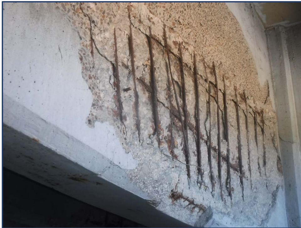
Photo 116-3 – Span 13, Active Corrosion on Maintenance Deck Stringers
