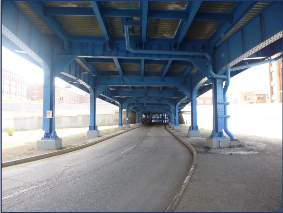
Unit IV Over West Lakeside Avenue Looking West
