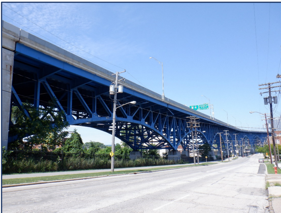
Unit II – Main Truss Span 1 Looking Northeast
