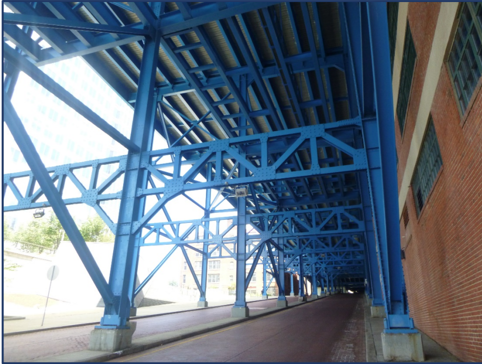
Unit III – Frame and Brace Typical Structure View Looking East
