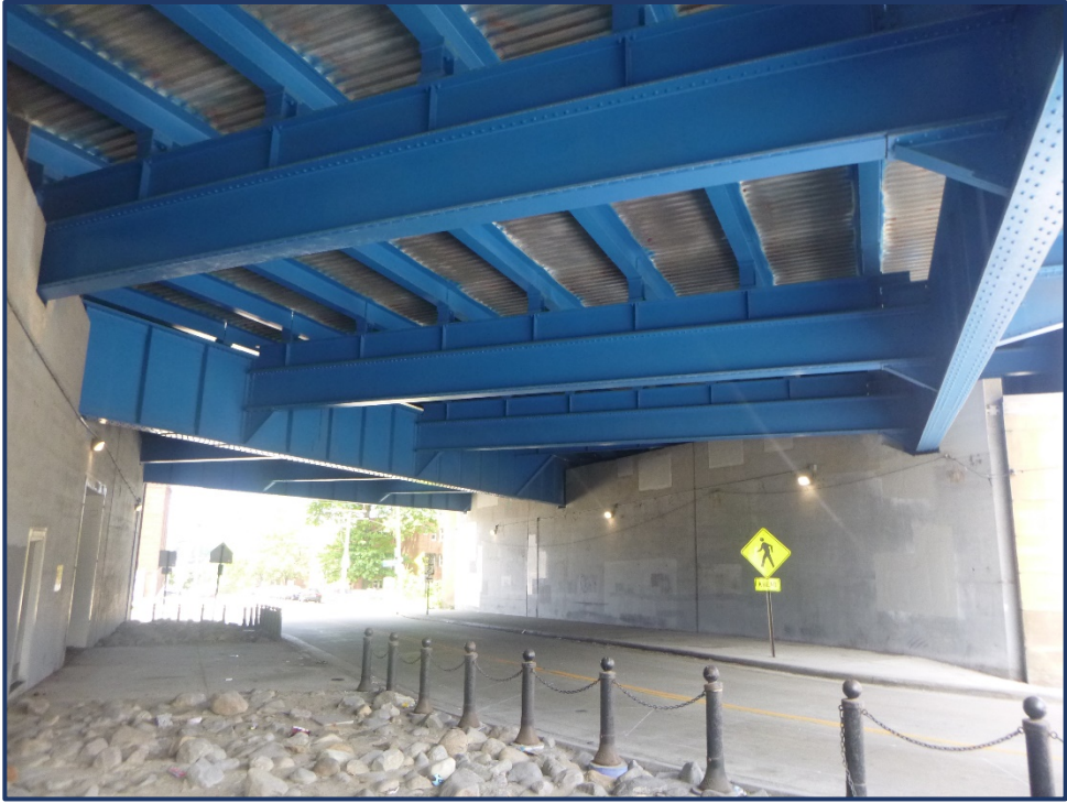
Section N Typical Superstructure Over W. 25 th Street Looking East
