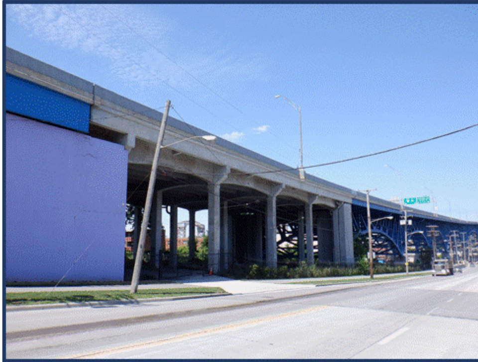
Section P Looking Northeast
