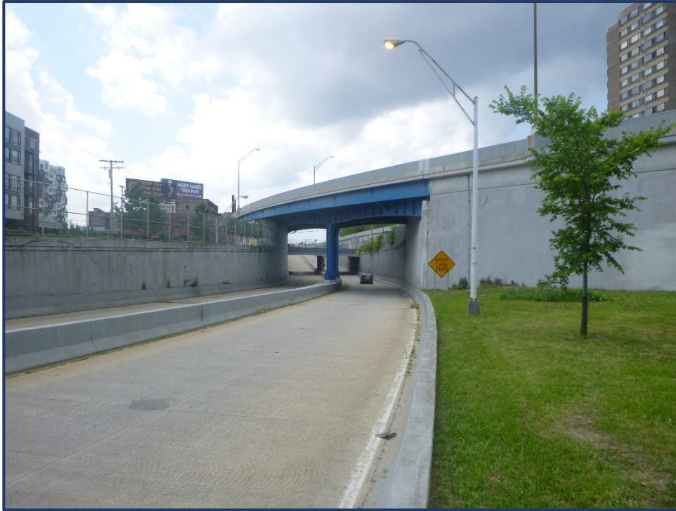
West 28 th Street Overpass Looking West
