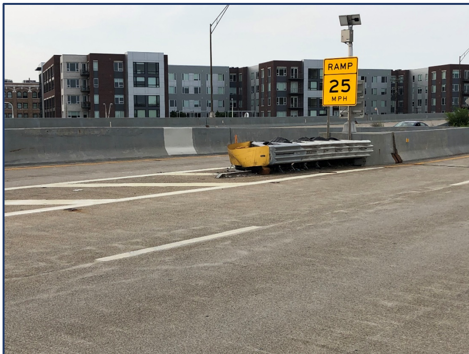
Photo APR-2 – Westbound Exist to W. 28 th St., Heavily Damaged Impact Attenuator
