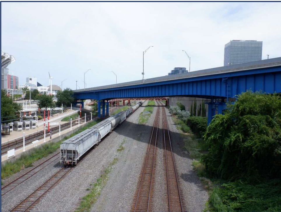
Unit V Lakefront Ramp Over CSX and NS Railroad Tracks Looking East
