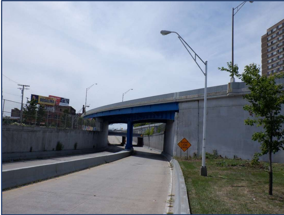
West 28 th Street Overpass Looking West
