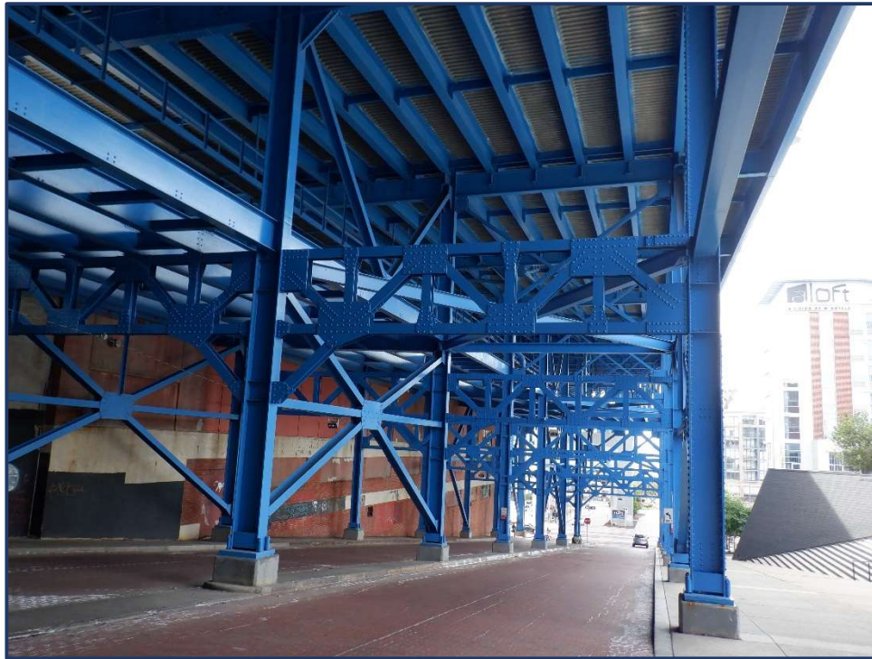
Unit III – Frame and Brace Typical Structure View Looking West
