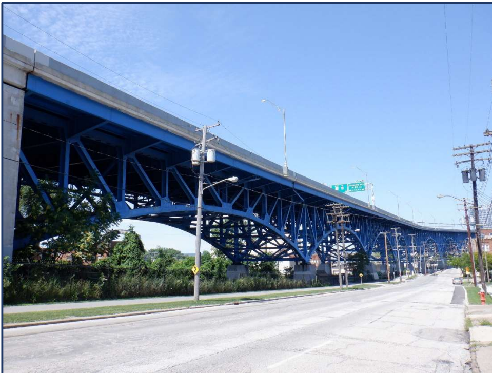
Unit II – Main Truss Span 1 Looking Northeast
