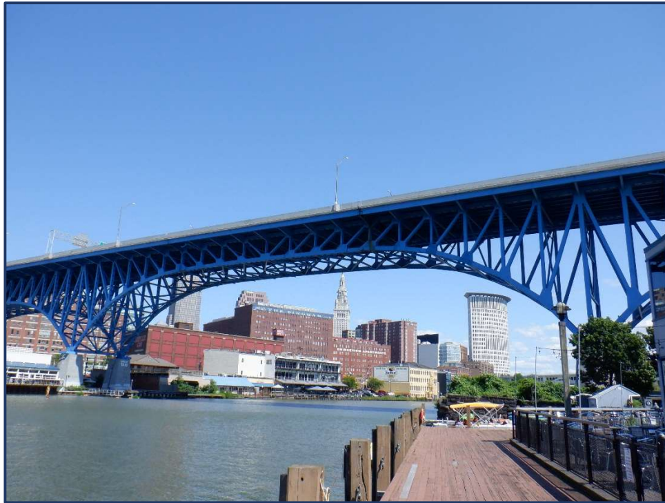
Unit II Span 9 Over the Cuyahoga River Looking South
