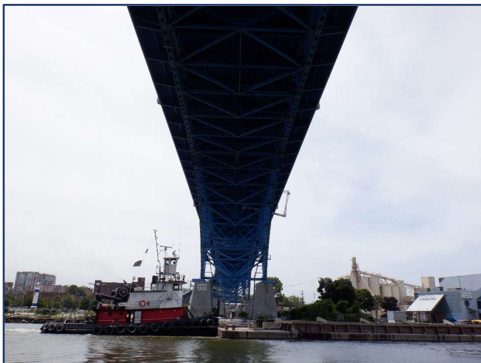
Unit II Span 9 Over the Cuyahoga River Typical Superstructure Looking West
