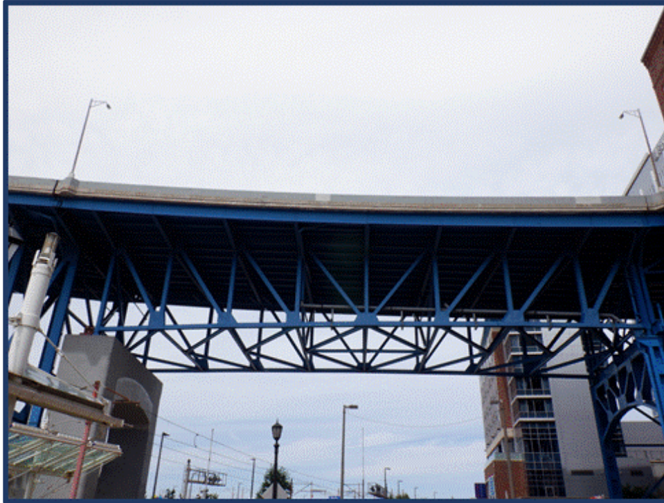
Unit III Span 11 Over West 10 th Street Looking North
