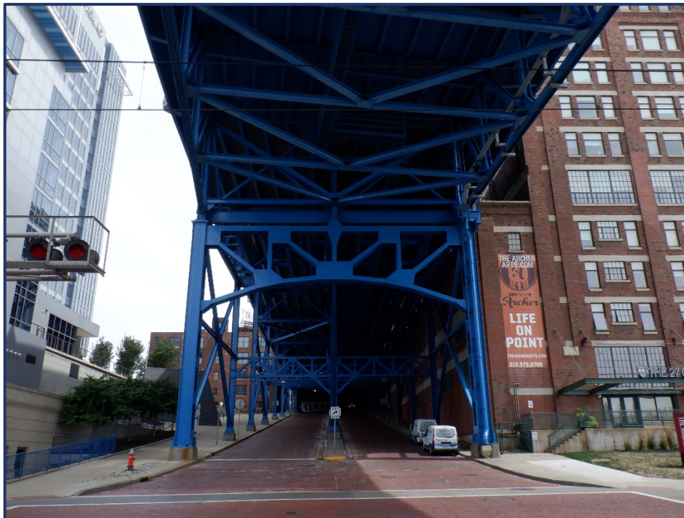
Unit III Bent 0 at West 10 th Street Looking East
