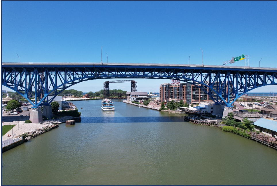
Unit II Span 9 Over the Cuyahoga River Looking South
