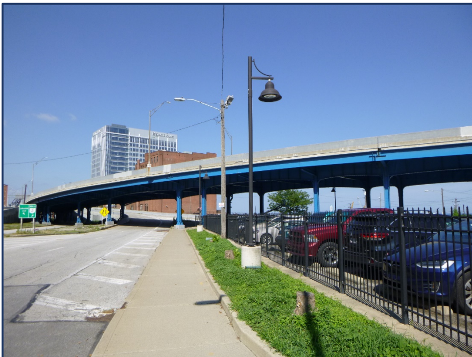
Unit IV South Elevation Over Ramp to SR-2 Westbound Looking Northwest
