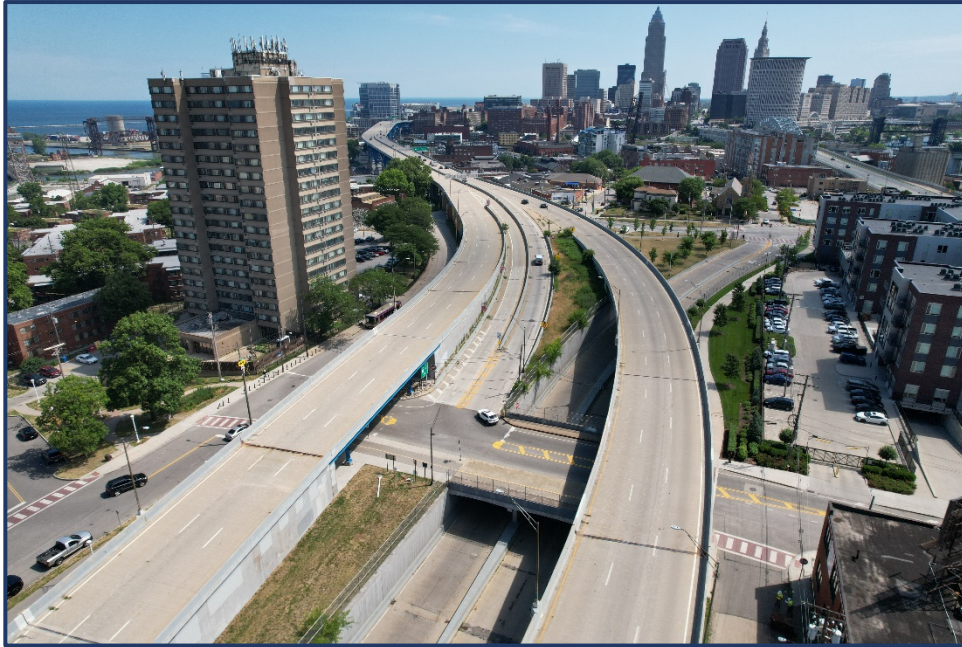
Unit I and II Deck Looking East
