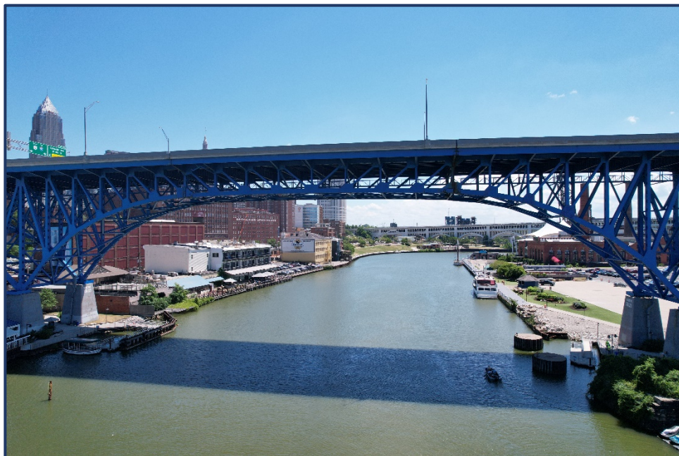
Photo CH-1 – Channel at Bridge Looking South
