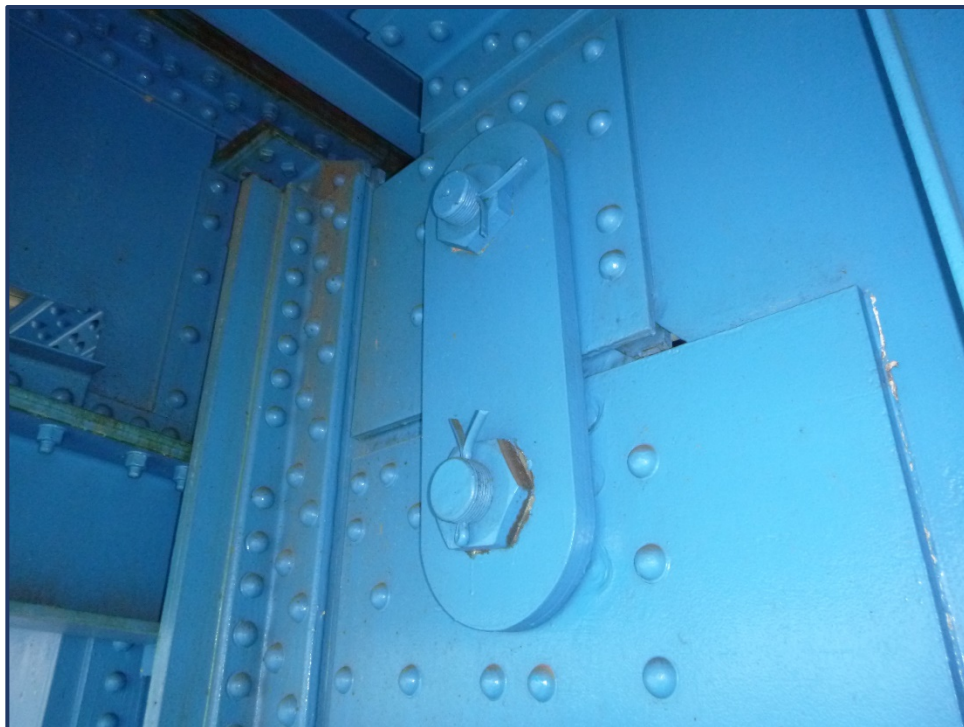
Photo 161-3 – Unit IV, Span E, Hanger Assembly Near Joint B4
