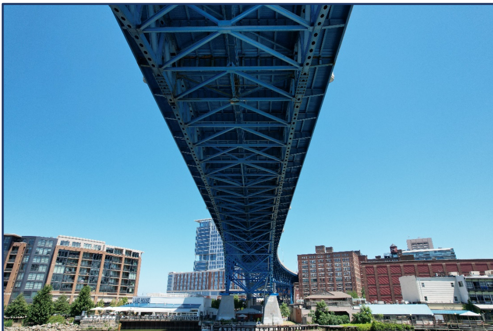
Unit II Span 8-10 Typical Superstructure Looking West
