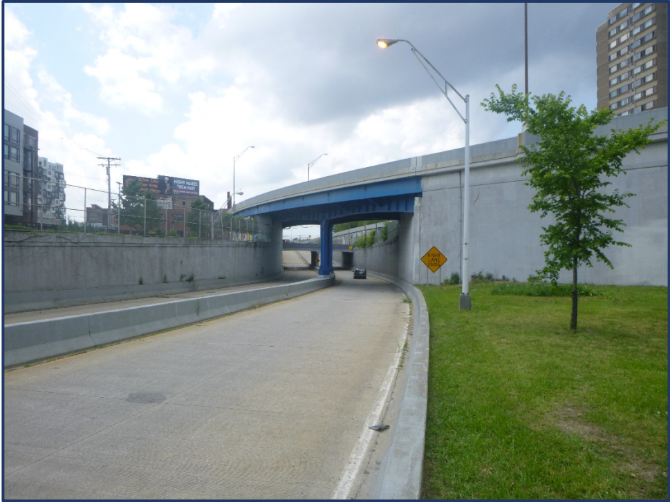
West 28 th Street Overpass Looking West
