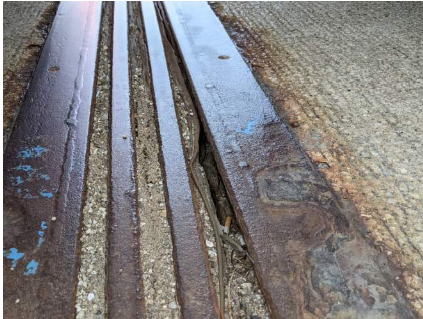
Photo 6: Assembly Joint with Seal with Splitting Seal
