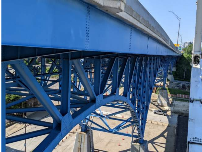
Photo 17: North Truss Elevation, Spans 1 Thru 3
