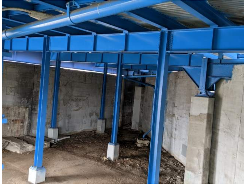
Photo 35: Steel Columns in Unit 1
