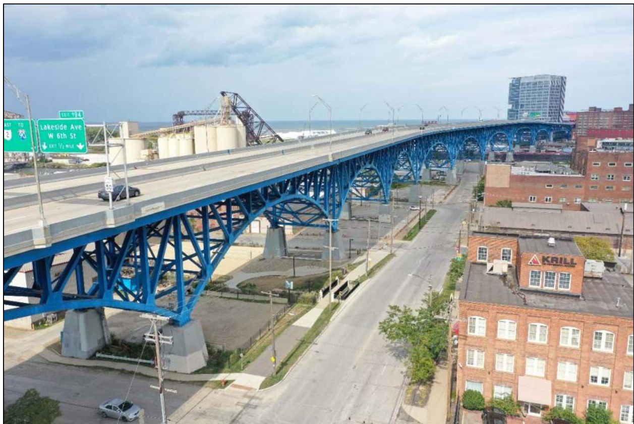
Figure 1: CUY-10-1613 over the Cuyahoga River
