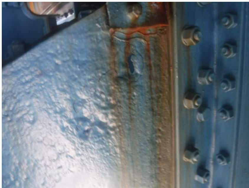
Photo 27: Upper Chord Outboard Gusset Plate at Span 7 North Truss, U6
