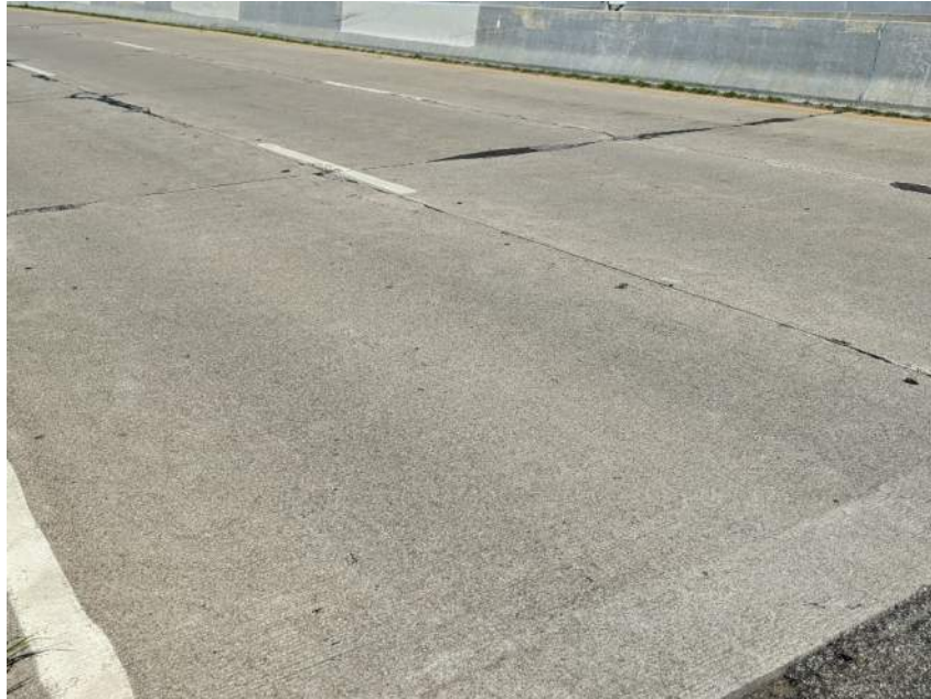
Photo 48: Typical Approach Wearing Surface
