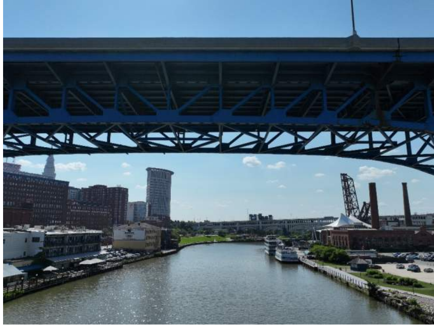
Photo 43: Channel at Bridge, Looking Upstream
