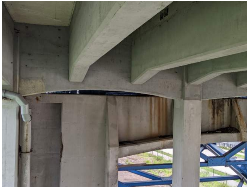
Photo 15: Reinforced Concrete Stringers, Unit I, Section P
