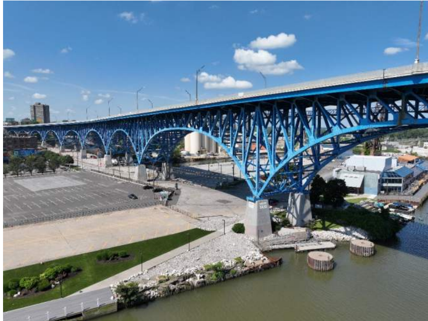
Photo 46: Channel Protection, West Bank
