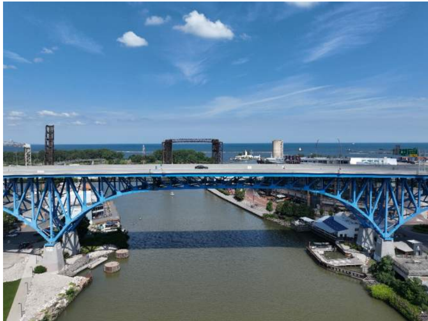
Photo 44: Channel at Bridge, Looking Downstream
