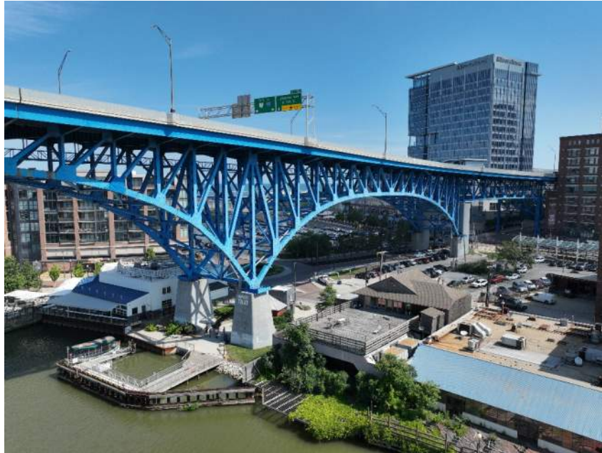
Photo 45: Channel Protection, East Bank
