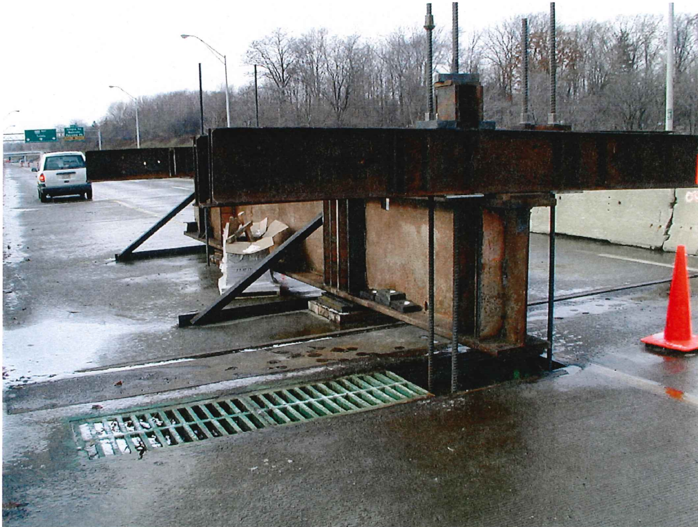
Picture 7 - Temporary Carrier Beam Installed Photo/ODOT
