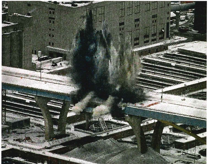
Picture 8 - Aerial View of the Hoan Bridge Demolition Photo/Gary Porter
