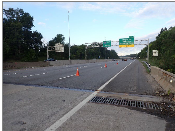
Photo 48 – Rear approach roadway resurfaced since the previous inspection, looking southwest.
