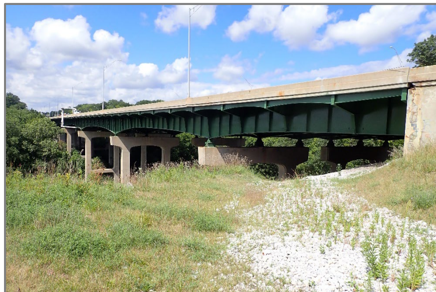
Figure 1 – CUY-480-0647 south elevation, looking northwest.
