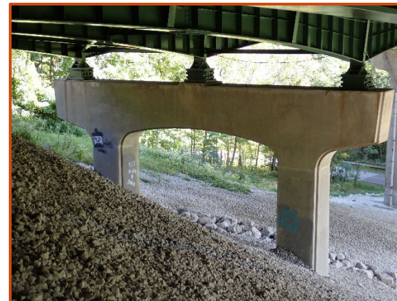
General view of Pier 1 for the westbound structure, looking east.
