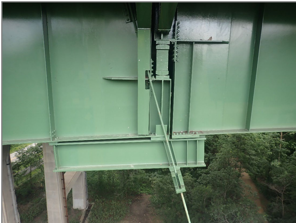
Photo 8 – Typical carrier beam retrofit installed below the seated hinge joints, looking north at Girder A at the Span 4 expansion joint.
