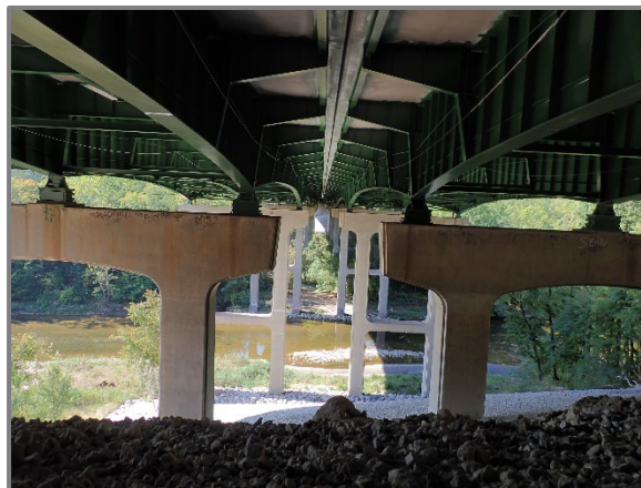
Photo 1 – Superstructure underside of the CUY-480-0647 Bridge, looking west from Forward Abutment.
