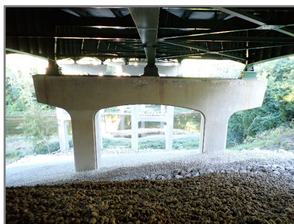
Photo 48 – View of slope protection on east slope from the Forward Abutment, looking west.
