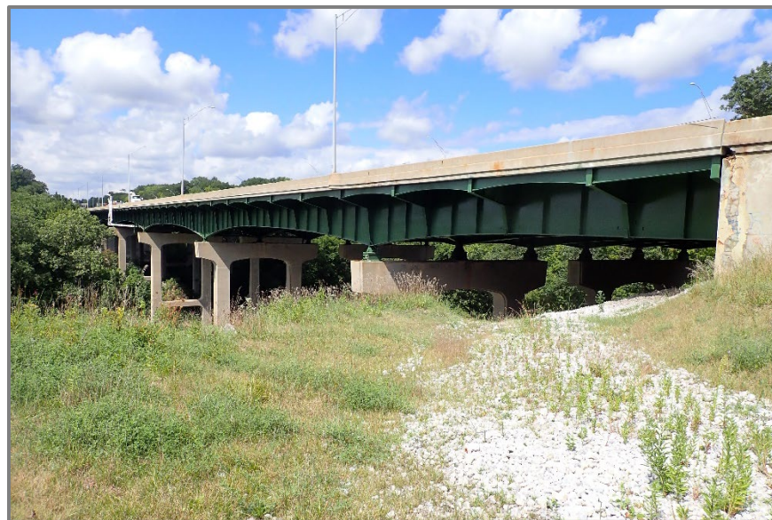
Figure 1 – CUY-480-0647 south elevation, looking northwest.
