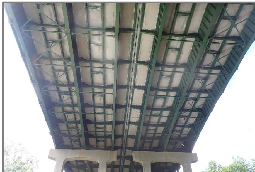
Figure 3 – CUY-480-0647 superstructure underside, looking west in Span 7.
