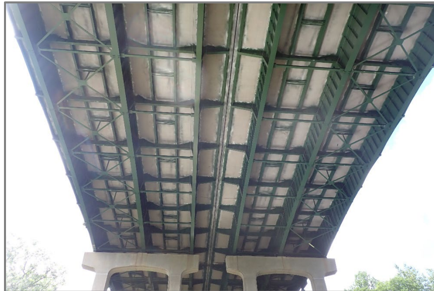
Figure 3 – CUY-480-0647 superstructure underside, looking west in Span 7.
