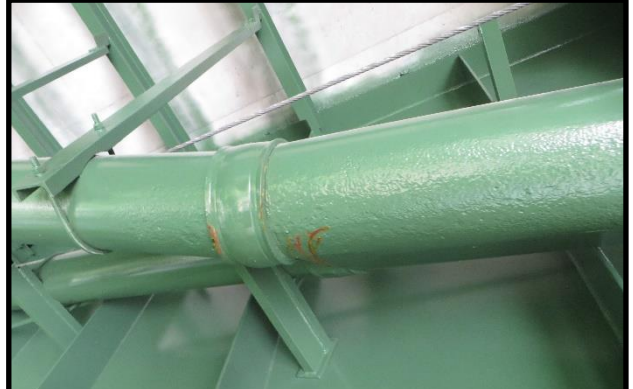
Photo 19 – Westbound Span 6 downspout 2021
