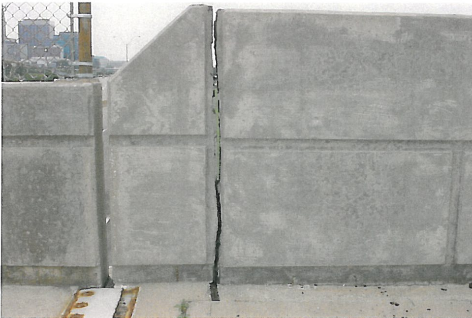
Photo #24 South Marginal Road bridge structure (Memorial Shoreway) – Northwest abutment
