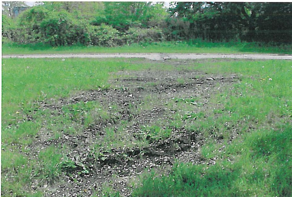
Photo #18 South Marginal Road – Area of previous trench work
