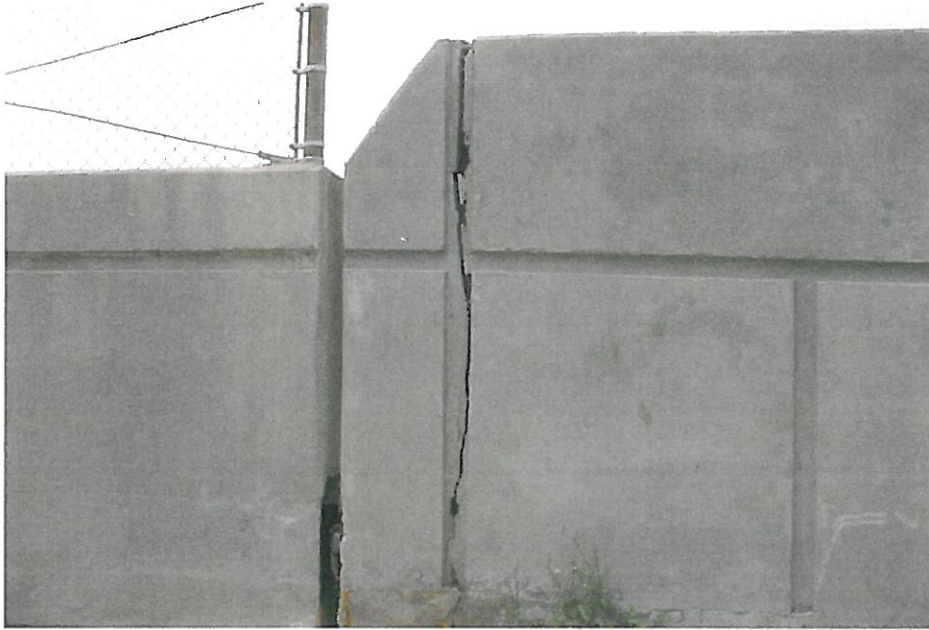
Photo #23 South Marginal Road bridge structure (Memorial Shoreway) – Northeast abutment
