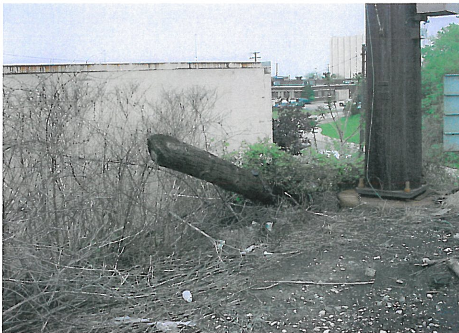
Photo #34 CSX Railroad bridge structure over East 55 th Street – Downed telephone pole
