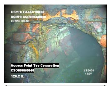
**Distance**: 120.2 ft. **Grade**: 0 **Condition**: Access Point Tee Connection
