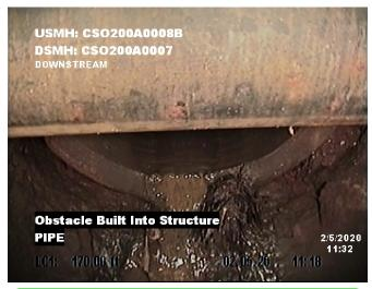
170.0 ft. Distance: Grade: 2 Condition: Obstacle Built Into Structure
