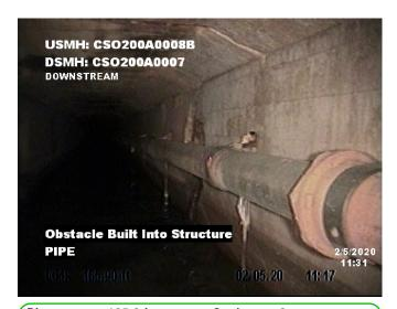
Distance: 165.9 ft. Grade: Condition: Obstacle Built Into Structure
