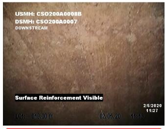
Distance: 18.0 ft. Grade: Condition: Surface Reinforcement Visible
