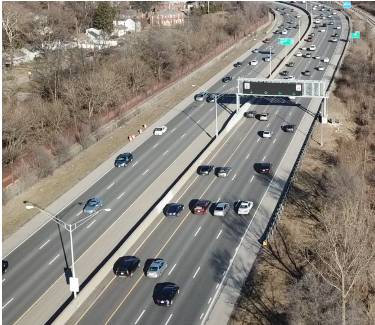
Figure 8 – SmartLane along I-670 EB in Columbus, Ohio
