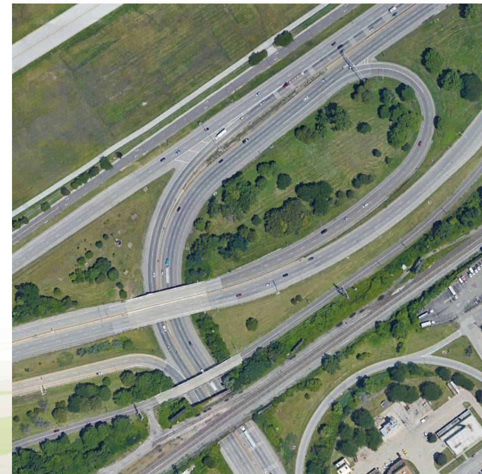
Figure 4 – I-90 through the SR 2 interchange
