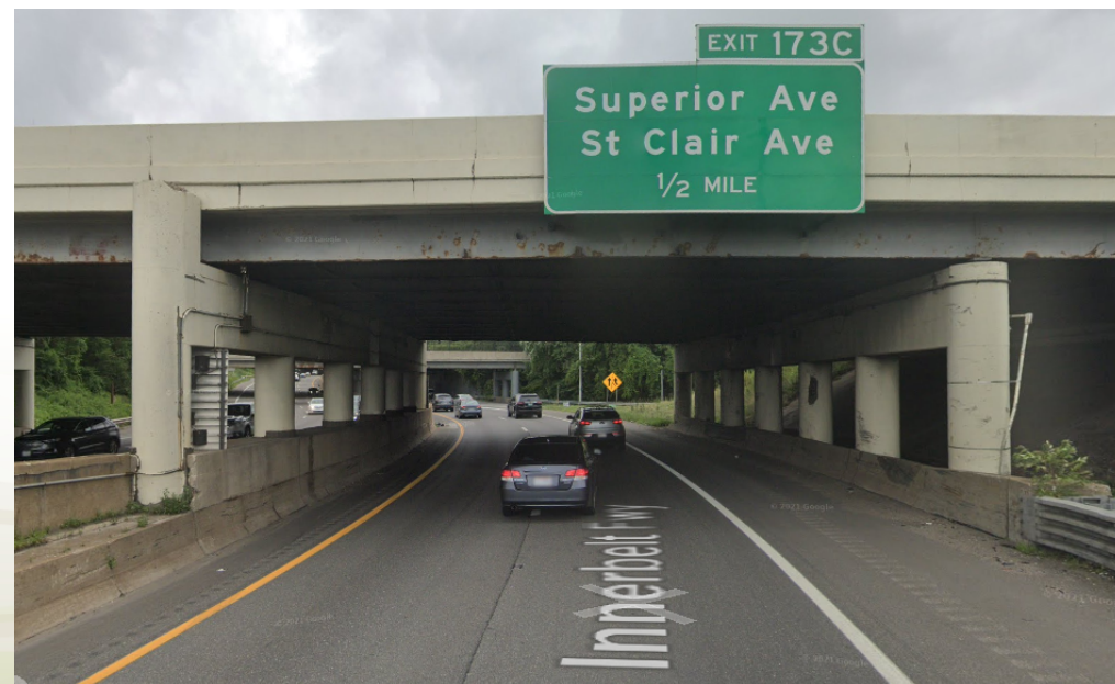
Figure 10 – Google Street View of I-90 WB traveling under the existing SR 2 Bridge
