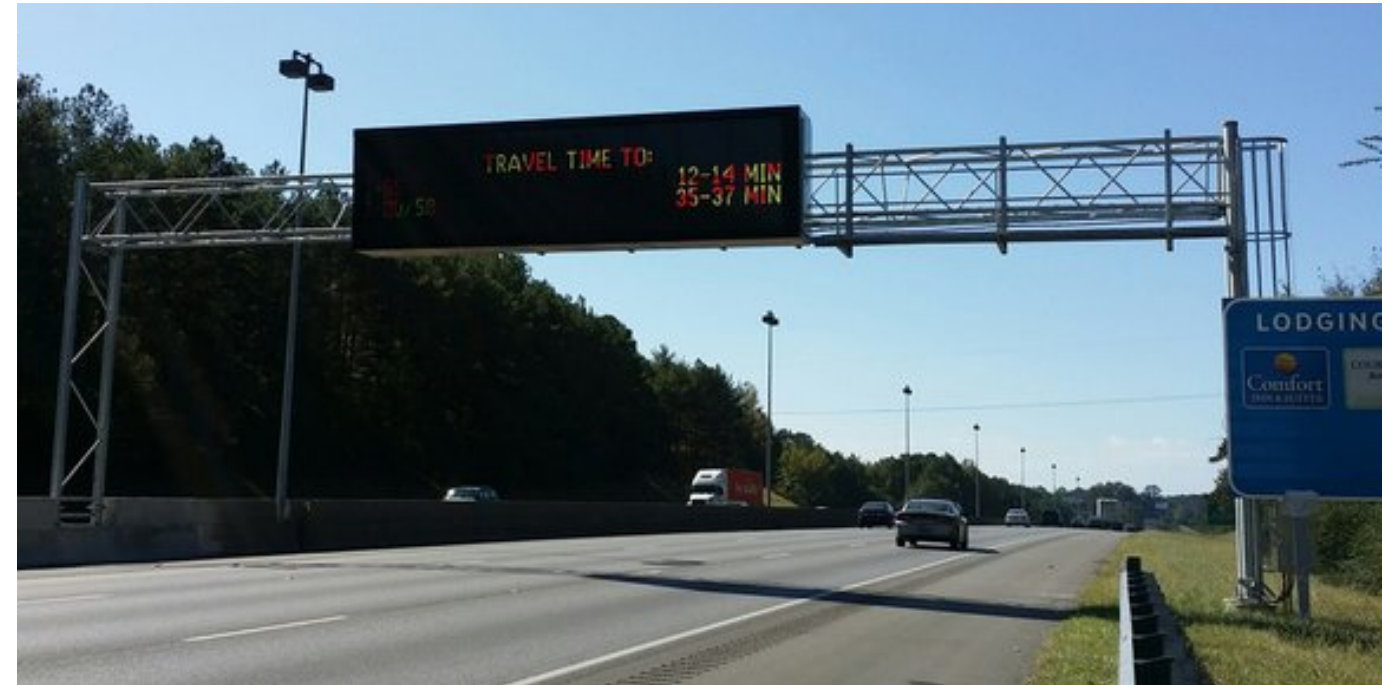
Figure 13 – Standard walk-in DMS
