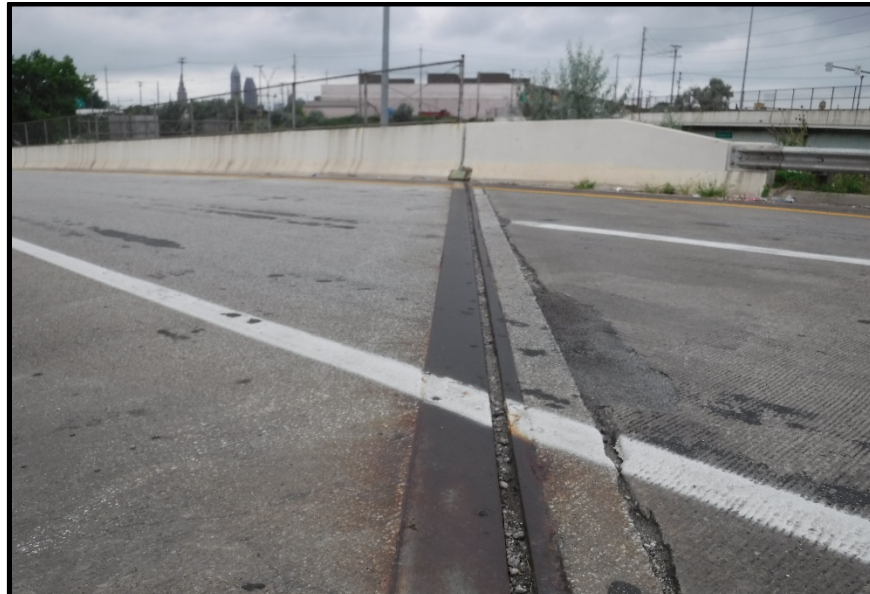
Photo 27 – Typical sliding plate joint in good condition
