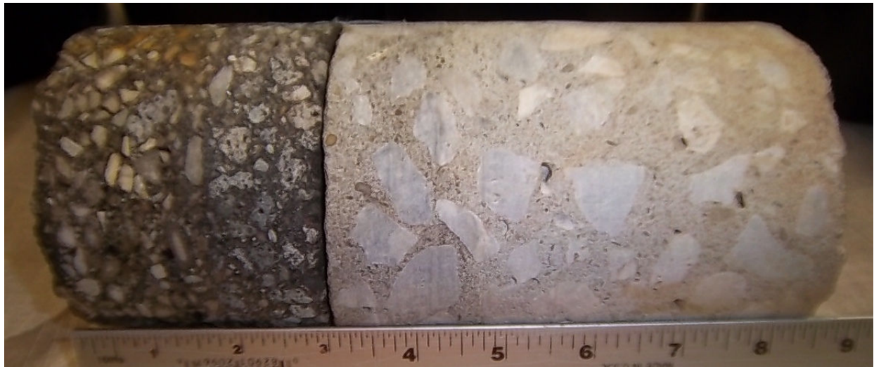
Core #49 Location: South Center of Intersection 3" Asphalt / 5 ½" Concrete
