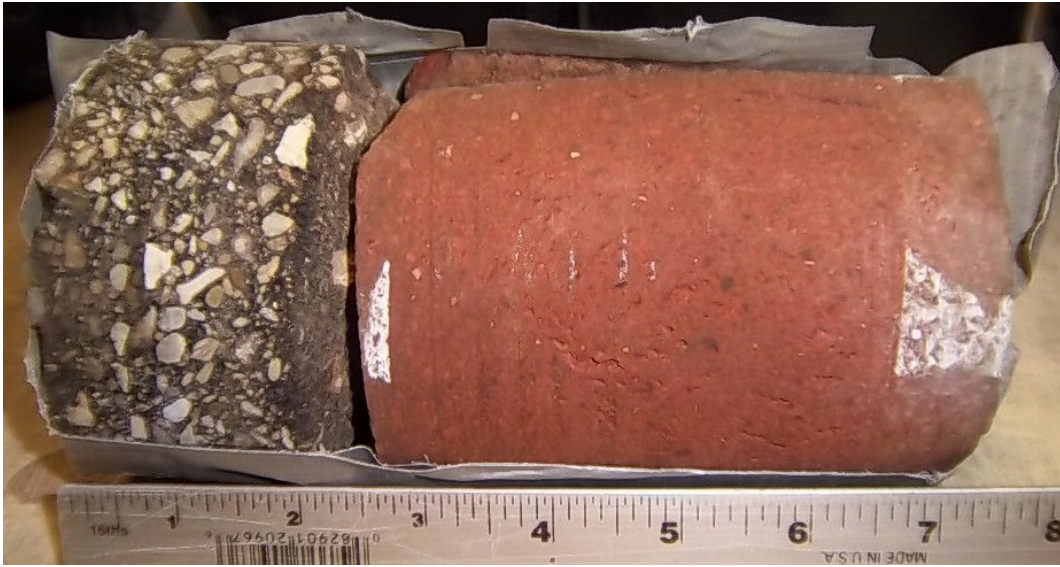
Core #51 Location: East Center of Intersection 2 ½" Asphalt / 4 ¾" Brick
