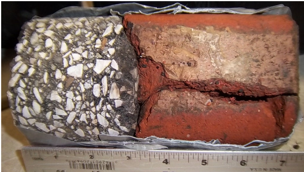
Core #46 Location: SW, South on W. 10 th St. 3" Asphalt / 4" Brick
