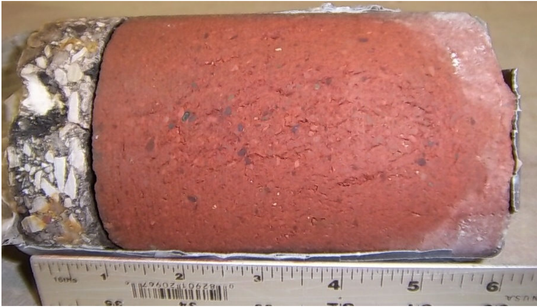
Core #53 Location: NE, North on W. 10 th St. 1" Asphalt / 5" Brick
