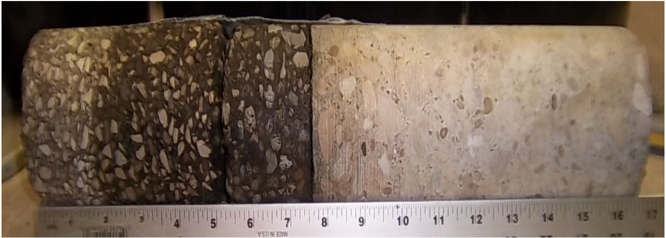
Core #47 Location: SW, Center on W. 10 th St. 7 ½" Asphalt / 9" Concrete
