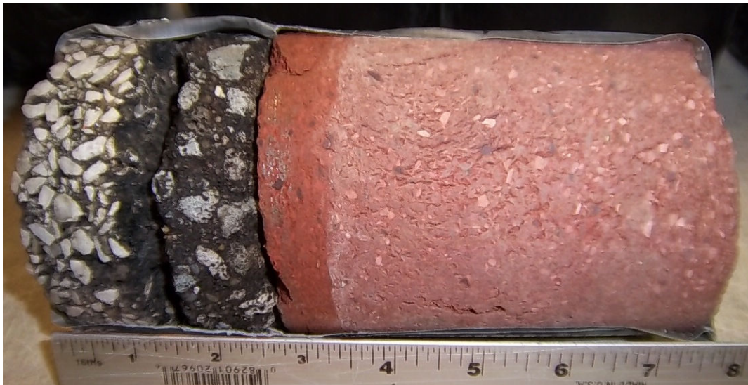
Core #52 Location: NE, East on W. 10 th St. 2 ½" Asphalt / 5" Brick
