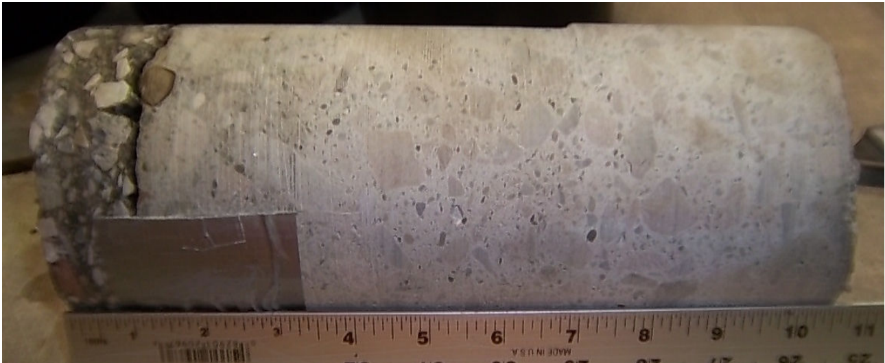
Core #44 Location: SE, Center on Professor Ave. 1" Asphalt / 9 1/2" Concrete
