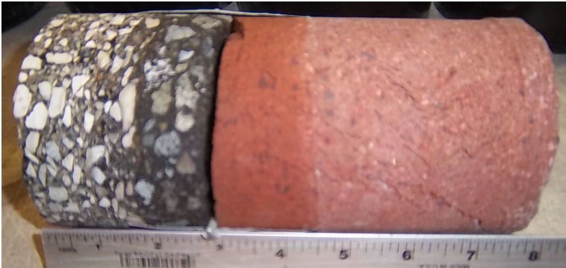
Core #48 Location: SW, West on W. 10 th St. 2 ¾" Asphalt / 5" Brick
