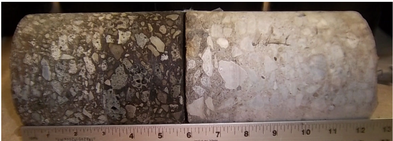
Core #50 Location: Center of Intersection 5 ¾" Asphalt / 6 ¾" Concrete
