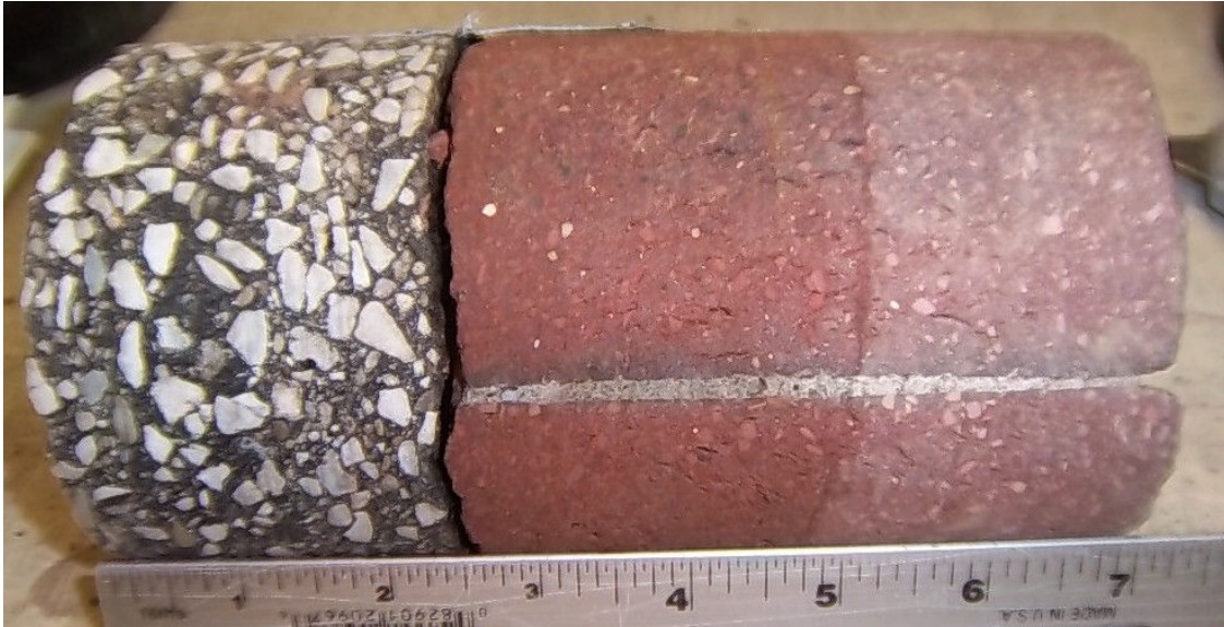
Core #34 Location: NW, North on Professor Ave. 2 ½" Asphalt / 4 ½" Brick
