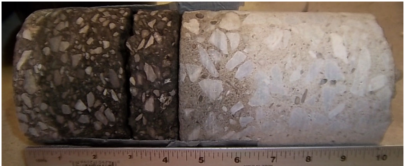
Core #27 Location: NE Center of Intersection 4 1/4" Asphalt / 5 3/4" Concrete
