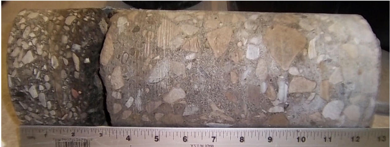
Core #30 Location: Center of Intersection 3" Asphalt / 9 1/2" Concrete
