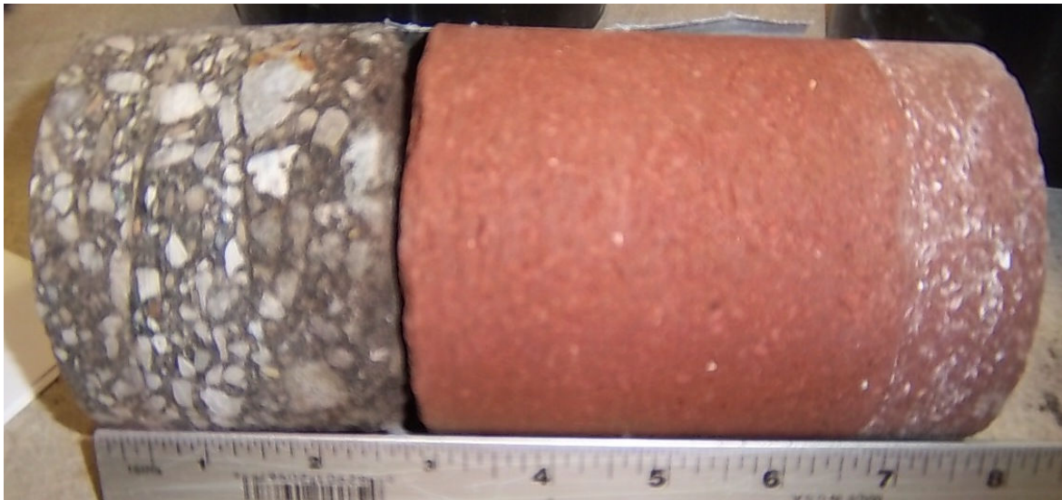
Core #31 Location: NE, North on Literary Ave. 2 3/4" Asphalt / 5 1/4" Brick
