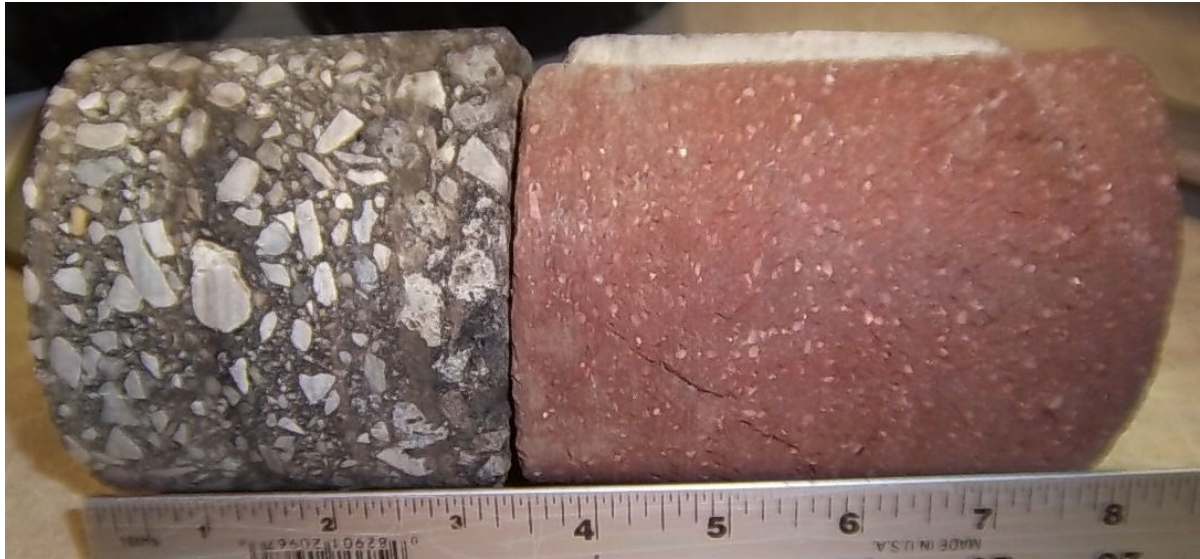
Core #38 Location: SW, Center on Literary Ave. 3 3/8" Asphalt / 4 1/2" Brick
