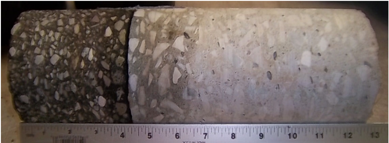
Core #40 Location: SE, South on Professor Ave. 4 ¼" Asphalt / 8" Concrete
