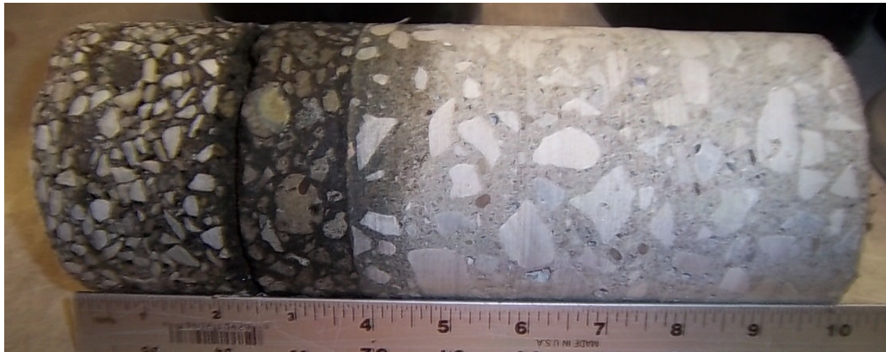
Core #29 Location: NW Center of Intersection 3 ¾" Asphalt / 6 ¼" Concrete
