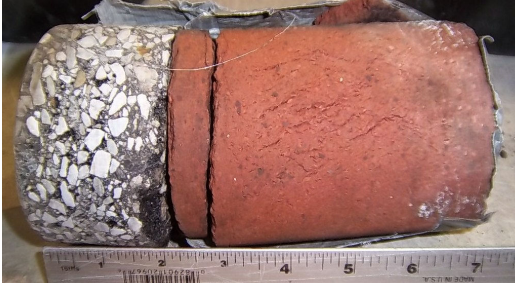
Core #36 Location: NW, West on Professor Ave. 2" Asphalt / 5" Brick
