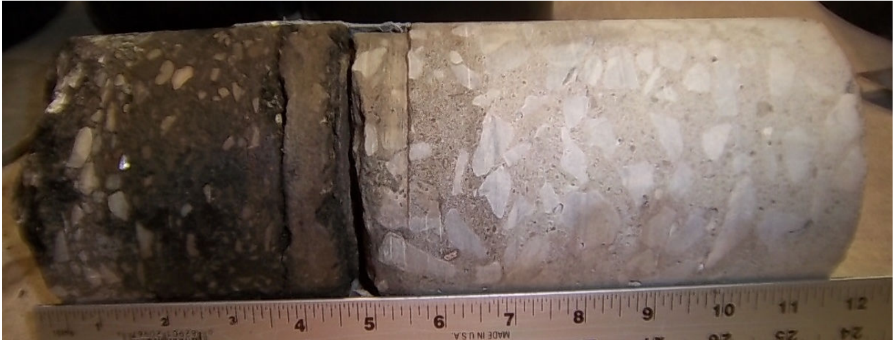
Core #42 Location: SE, East on Professor Ave. 4 3 / 4 " Asphalt / 6 3 / 4 " Concrete
