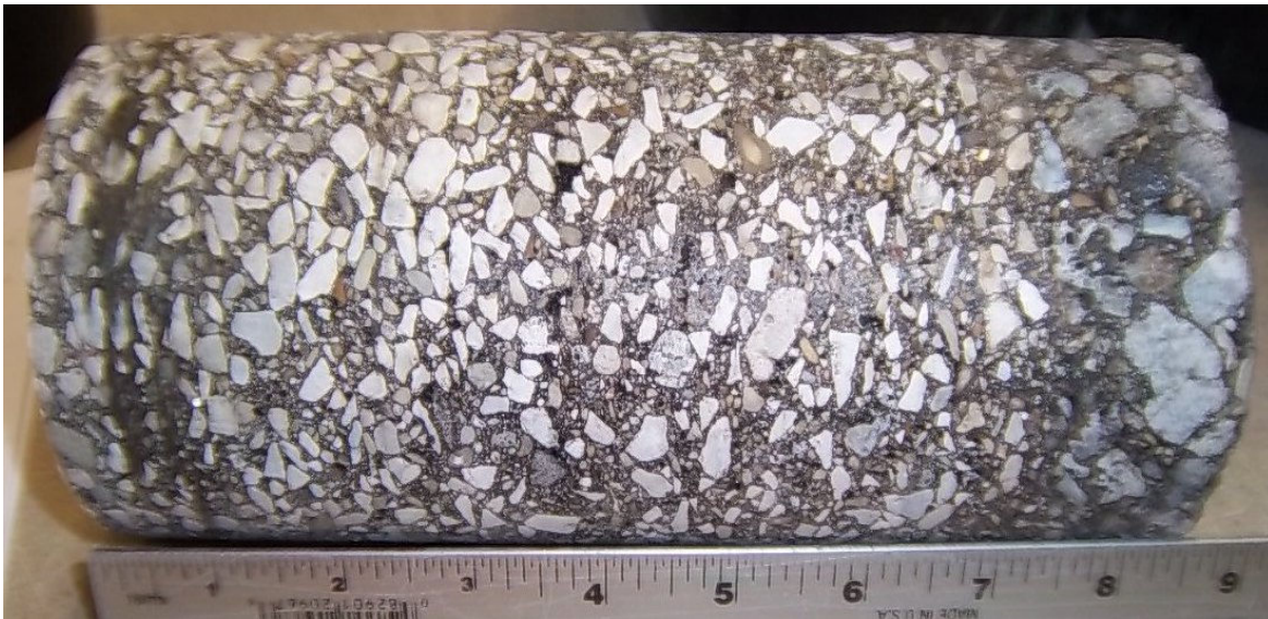
Core #24 Location: NW, Center on Professor Ave. 8 ½" Asphalt
