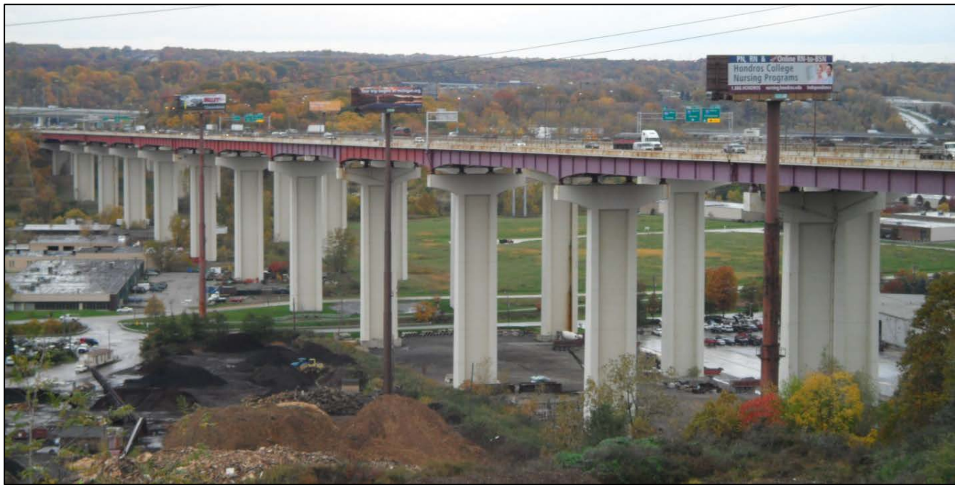
Picture #1 – General view looking northwest.
