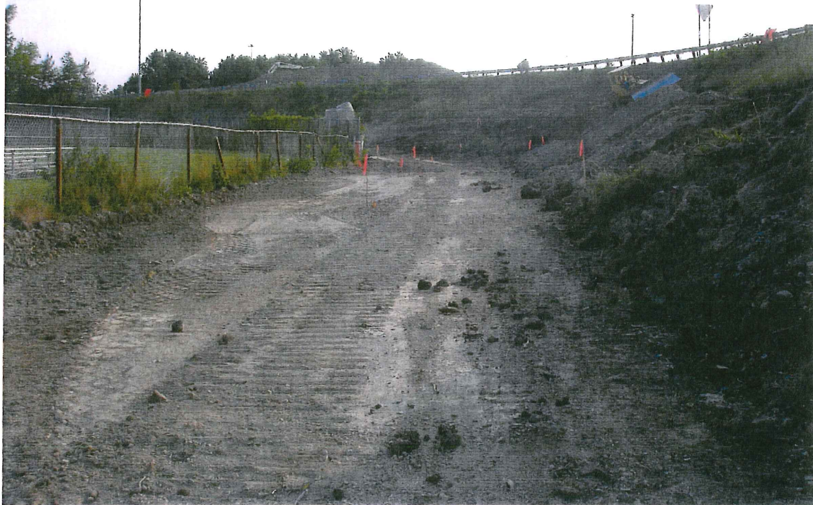
Photograph 1: View looking east along the proposed location of MSE wall.
