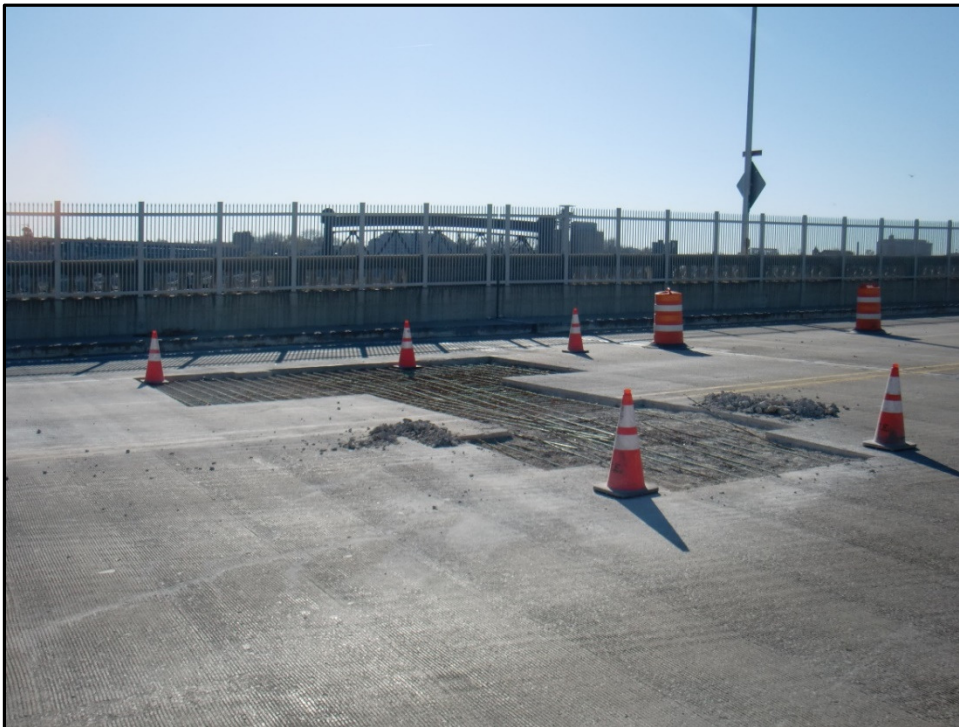
Photo 6 – Recent Wearing Surface Repair, Span 9 (November 2015).
