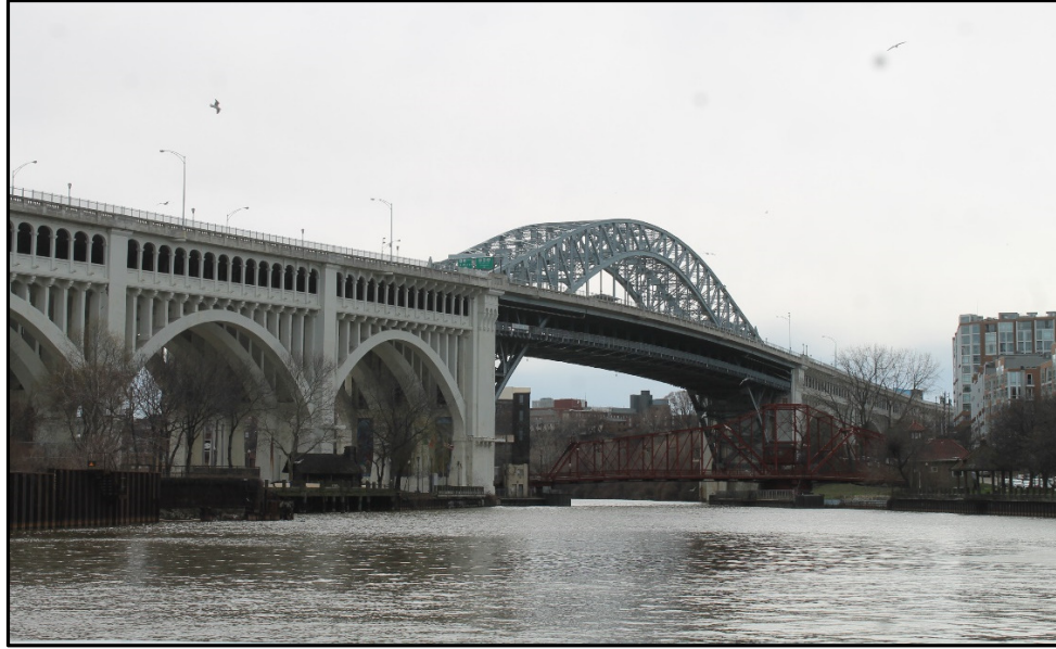
Photo 1– North Elevation, Spans 4 through 6.
