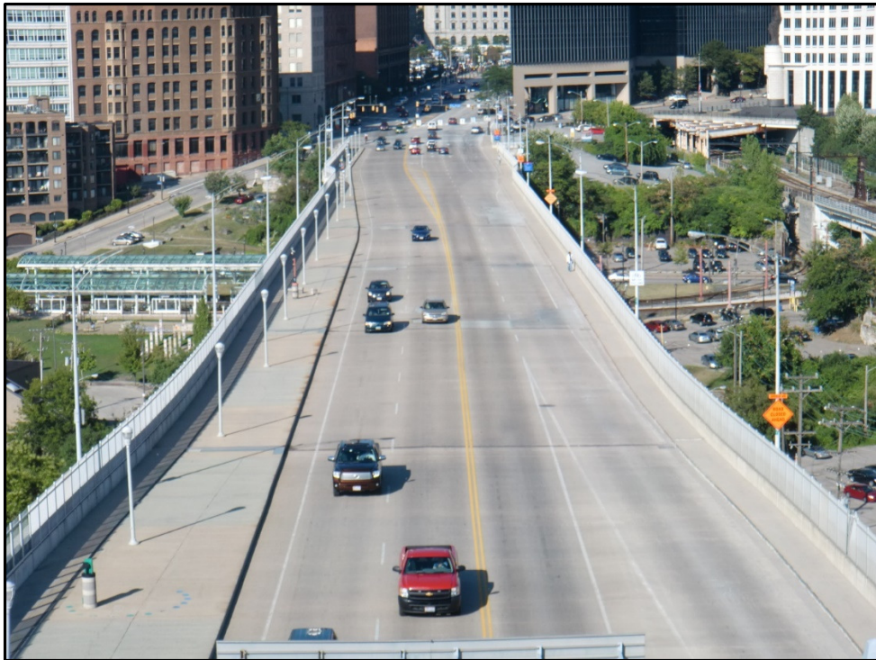
Photo 2– East Approach Spans Deck, Looking East.
