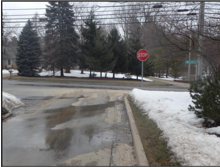
Looking north on Creekside Terrace toward the Wallings Road intersection
