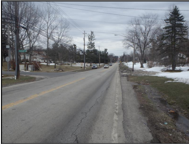
Looking east on Wallings Road toward the McCreary Road intersection
