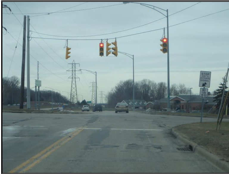
Looking north on Mill Road toward the Wallings Road intersection
