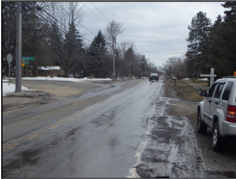
Looking west on Wallings Road toward the Creekside Terrace intersection
