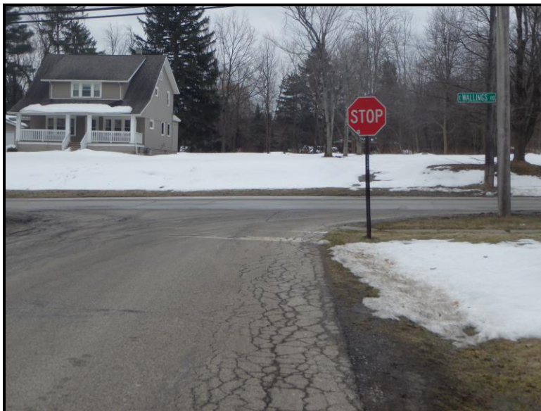
Looking south on Elmhurst Drive toward the Wallings Road intersection
