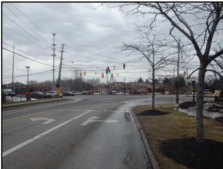
Looking east on Wallings Road toward the Broadview Road intersection
