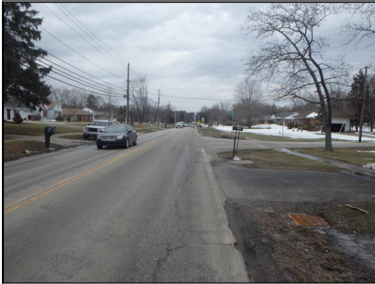
Looking east on Wallings Road toward the Chestnut Boulevard intersection
