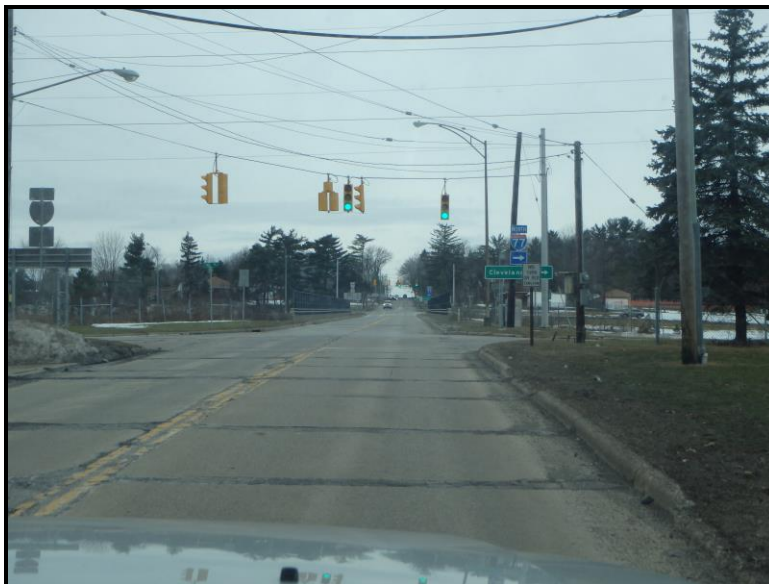
Looking west on Wallings Road toward the Mill Road / I-77 NB Entrance Ramp intersection
