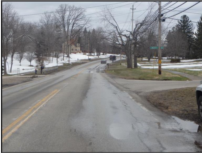
Looking west on Wallings Road toward the Longview Road intersection
