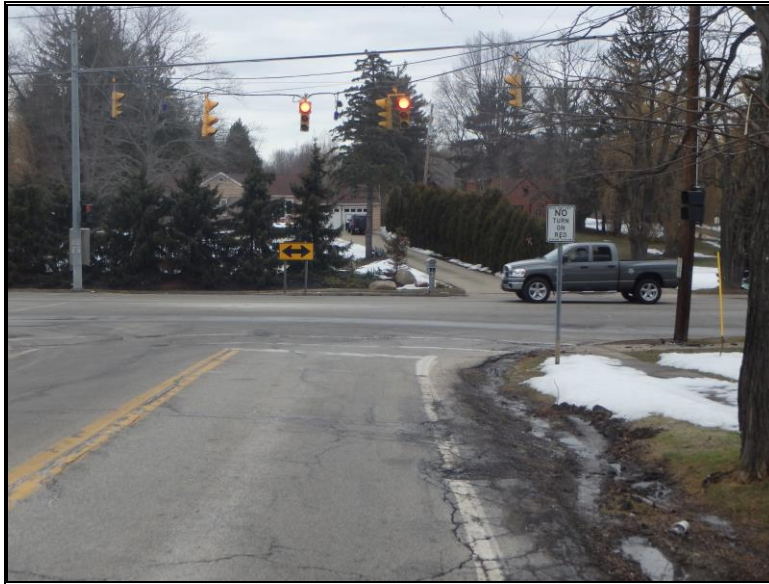
Looking north on Wyatt Road toward the Wallings Road intersection
