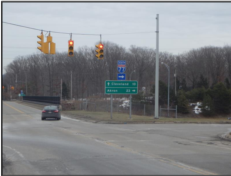
Looking east on Wallings Road toward the I-77 SB Ramps intersection
