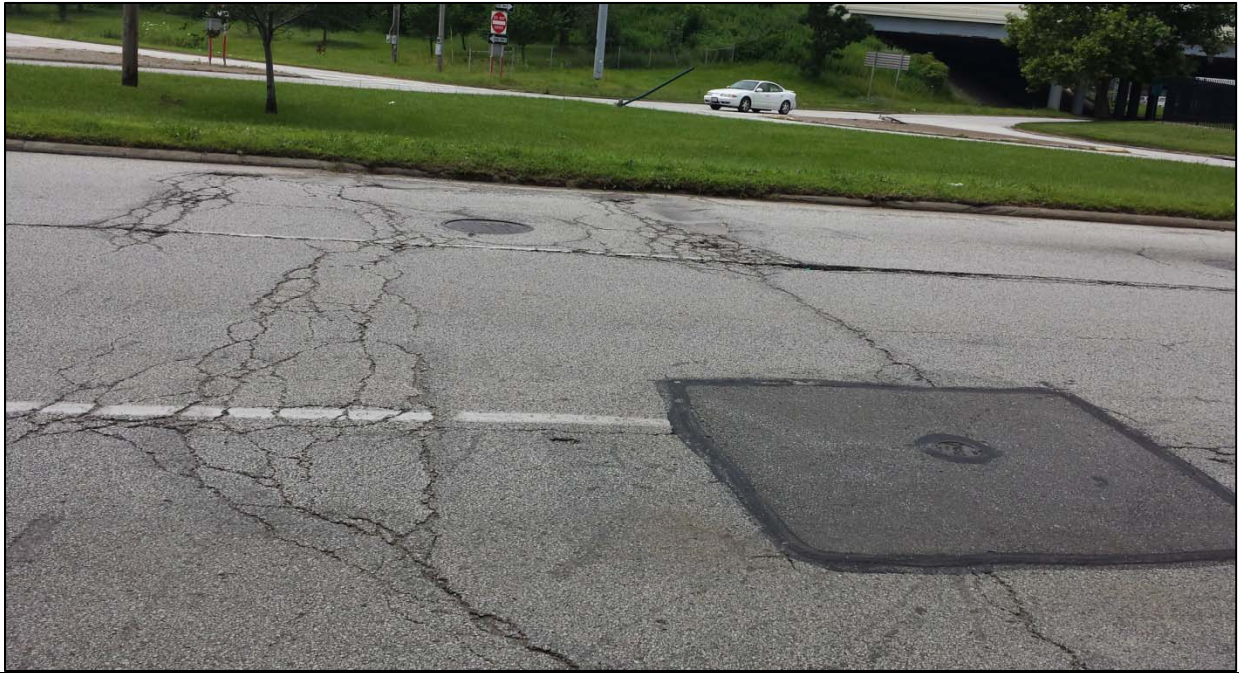
Photograph 8: East 22nd Street Pavement Distress
