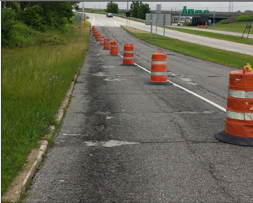
Photograph 4: Ramp H6 Pavement Distress Along Shoulder
