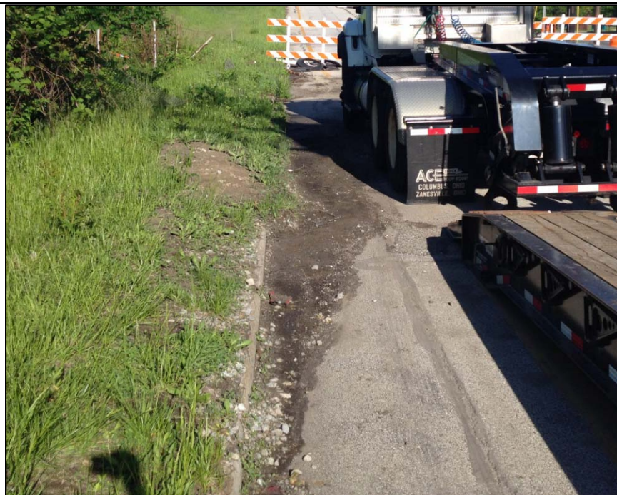
Photograph 2: Ramp H3 Poorly Drained Shoulder
