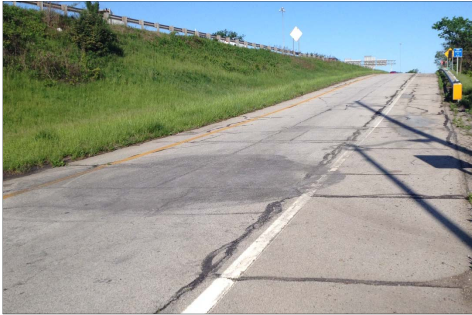
Photograph 2: Ramp H3 Poorly Drained Shoulder
