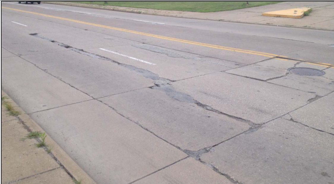
Photograph 6: East 30th Street Pavement Distress
