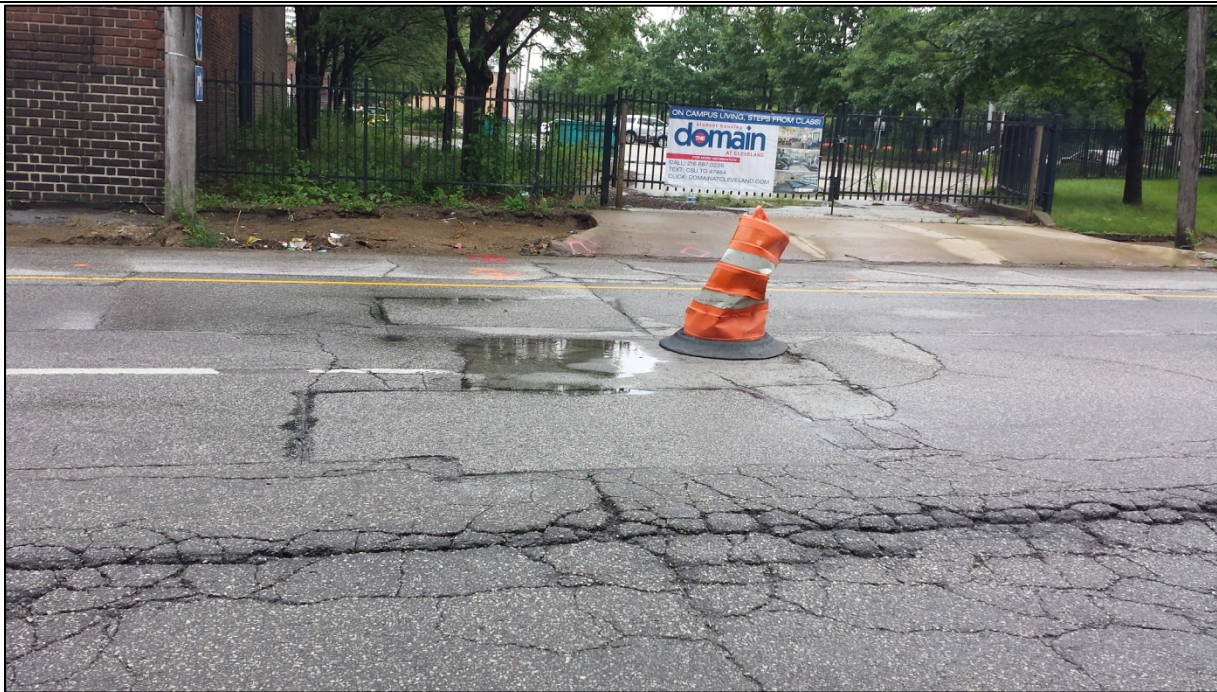
Photograph 8: East 22nd Street Pavement Distress
