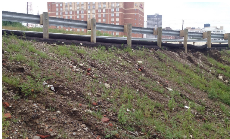
Photograph 5: Embankment erosion along Ramp A2 proposed alignment.
