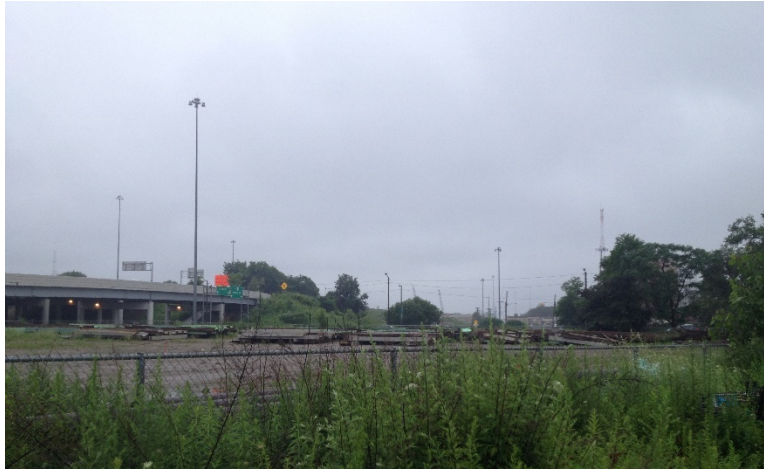
Photograph 4: Existing Ramp A2 bridge over abandoned ramp alignment.
