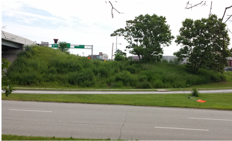
Photograph 3: IR-90 eastbound and supporting embankment slope
