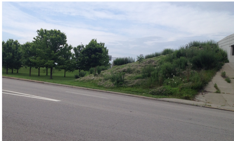
Photograph 1: Existing rear abutment spill-through slope
