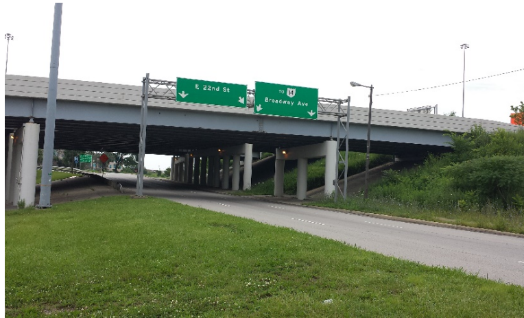
Photograph 3: Rear abutment spill-through/embankment slopes
