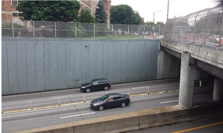
Photograph 2: Existing rear abutment west wing wall and slope
