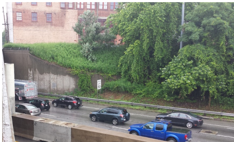
Photograph 1: Existing rear abutment wing wall and slope
