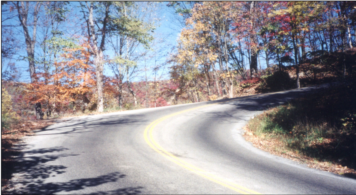
Rosemount Road - Excessive horizontal curves and steep grades make this route undesirable for truck traffic and impassable in severe weather.
