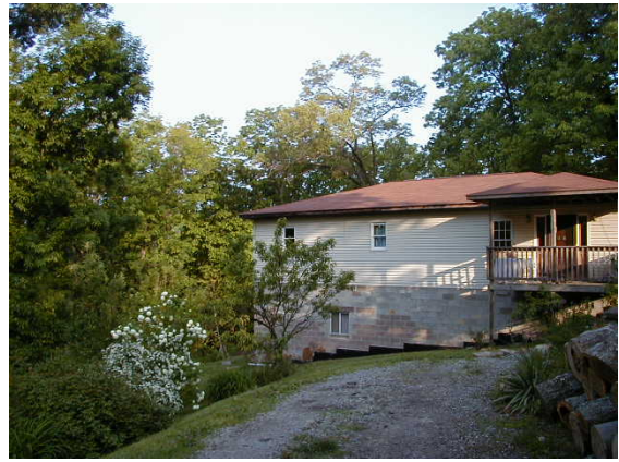
House used for receptor H2.
