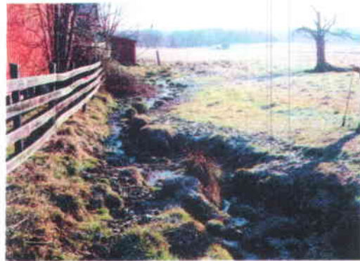
W14 WL6, emergent groundwater/surface water -fed wetland through active pasture adjacent to SR 335.
