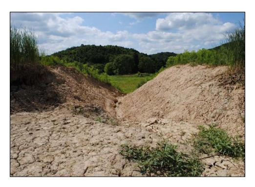
Photograph 11. View of breached berm at Wetland 7 (former Pond 3), facing northwest.
