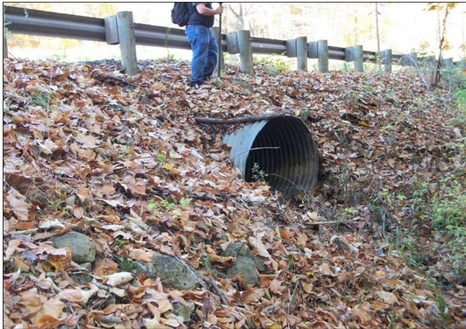
Photograph 306. Stormwater culvert at Stream 46 just south of Webster Street, facing north.
