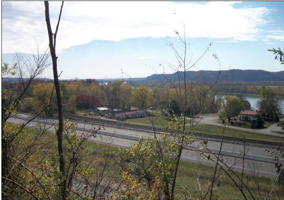
Photograph 314. Southern portion of corridor, overlooking US 52 and the Ohio River, facing southeast.
