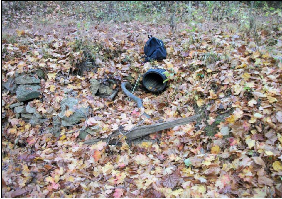
Photograph 301. Pipe from Stream 43 entering Stream 44, facing northeast.
