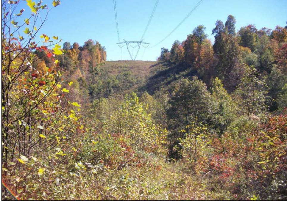
Photograph 225. Power line corridor, facing southeast.
