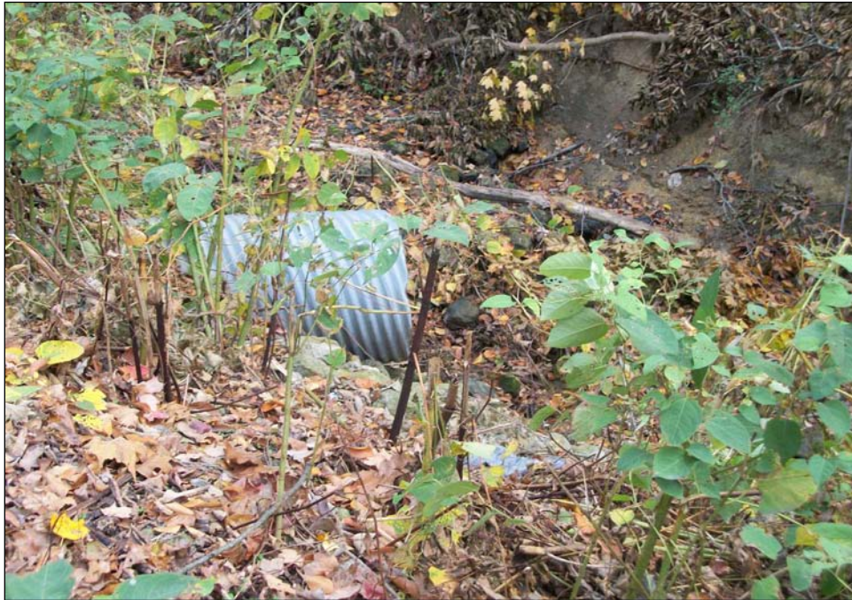
Photograph 312. Culvert from PJD 1 under SR 140/Webster Street to Stream 46.
