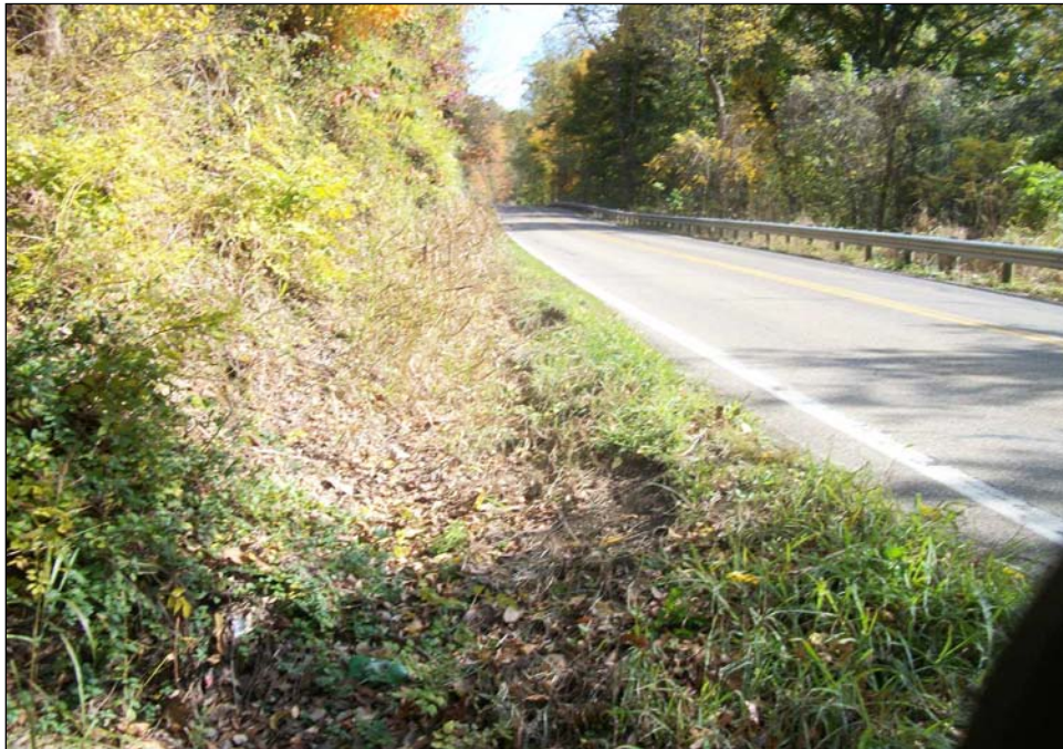
Photograph 254. Non-jurisdictional roadside ditch, facing east.
