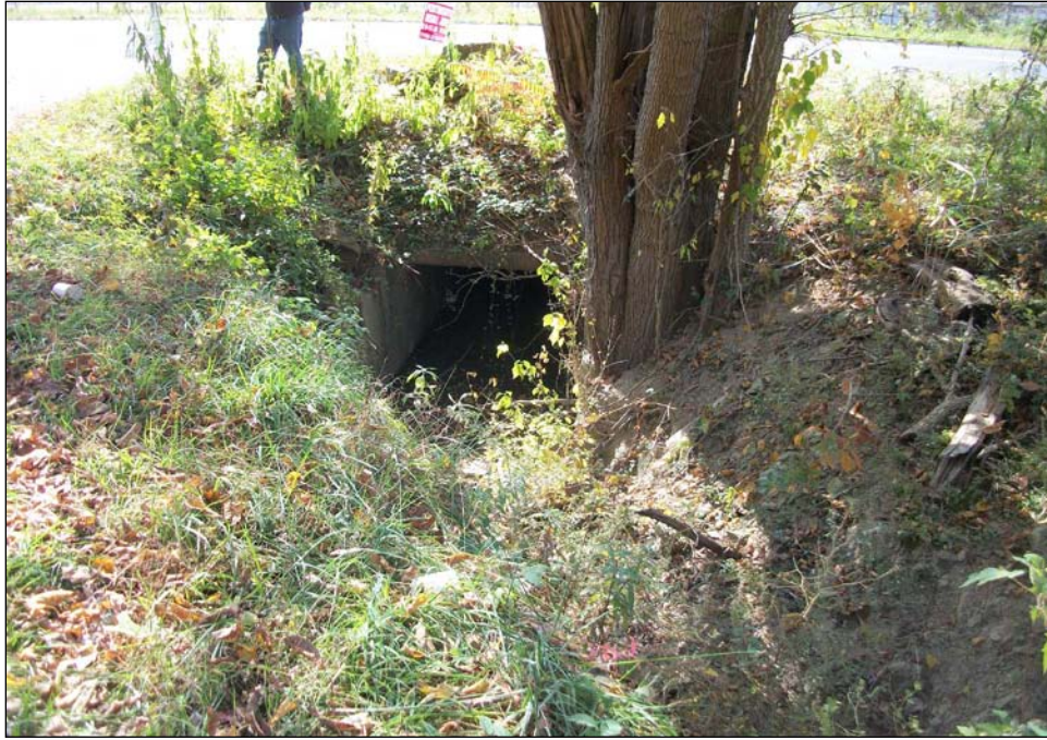
Photograph 317. Stream 47 culvert under Gallia Street, facing downstream (southwest).
