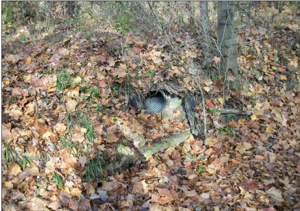
Photograph 304. Pipe from Stream 45 entering Stream 44 facing upstream (northwest).
