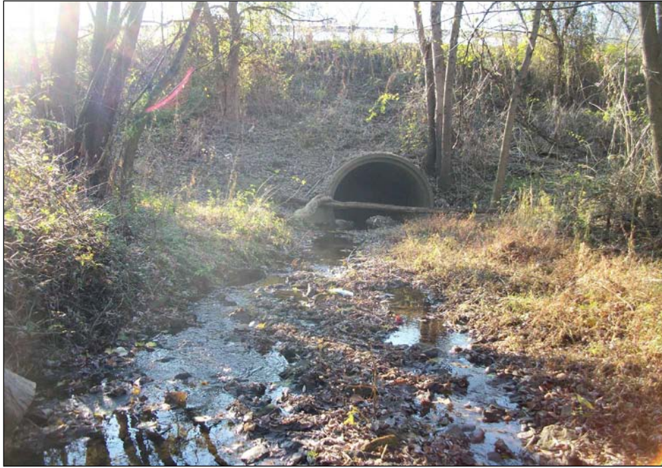
Photograph 325. Stream 48 culvert under US 52, facing downstream (southwest).
