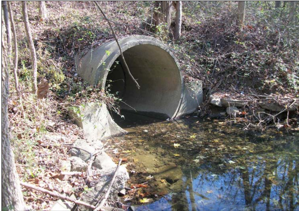
Photograph 324. Stream 48 culvert under US 52, facing upstream (northeast).
