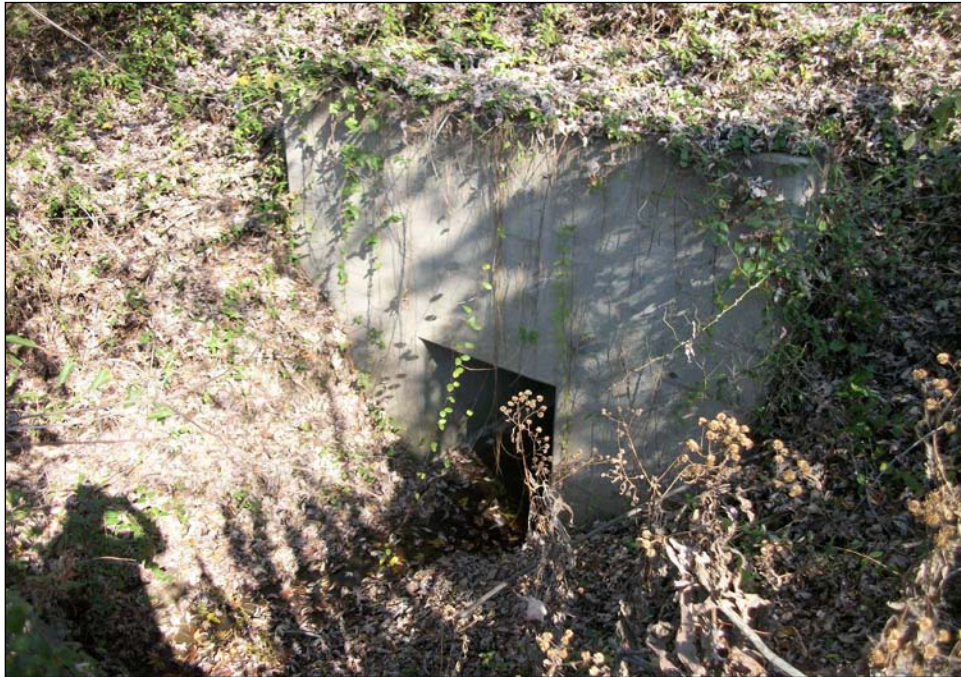
Photograph 318. Stream 47 culvert, facing northeast.
