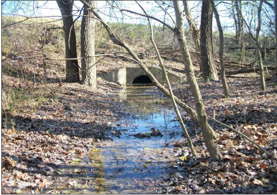
Photograph 327. Stream 49 culvert under US 52, facing upstream (east-southeast).
