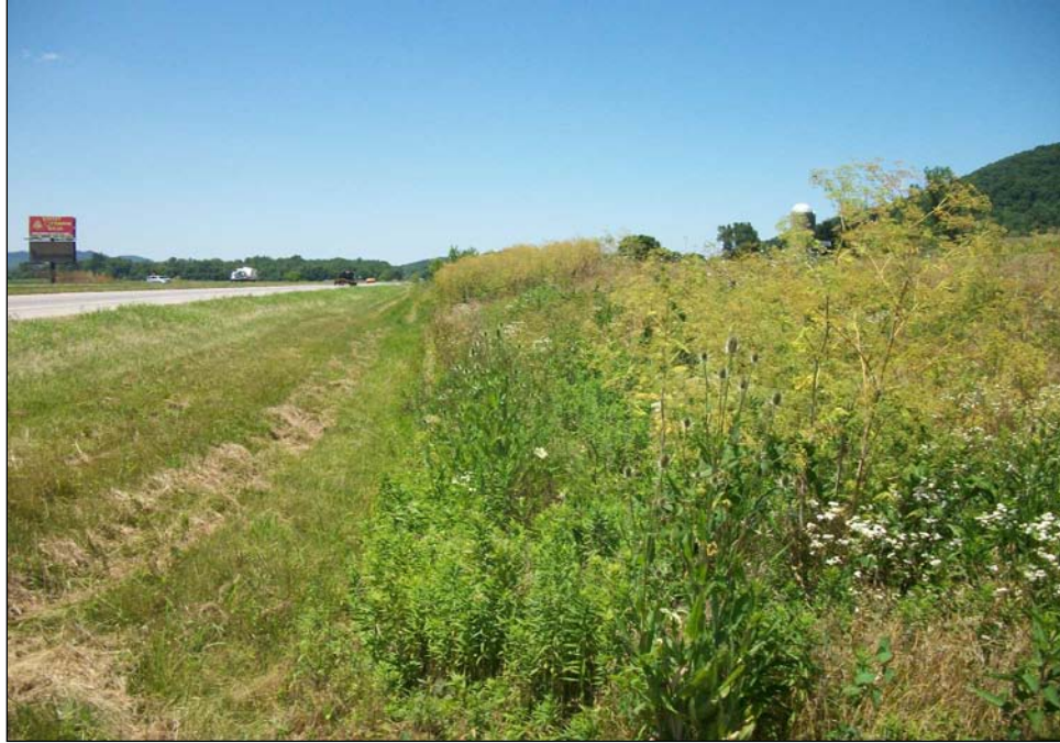
Photograph 19. Roadside ditch along US 23, facing northwest.
