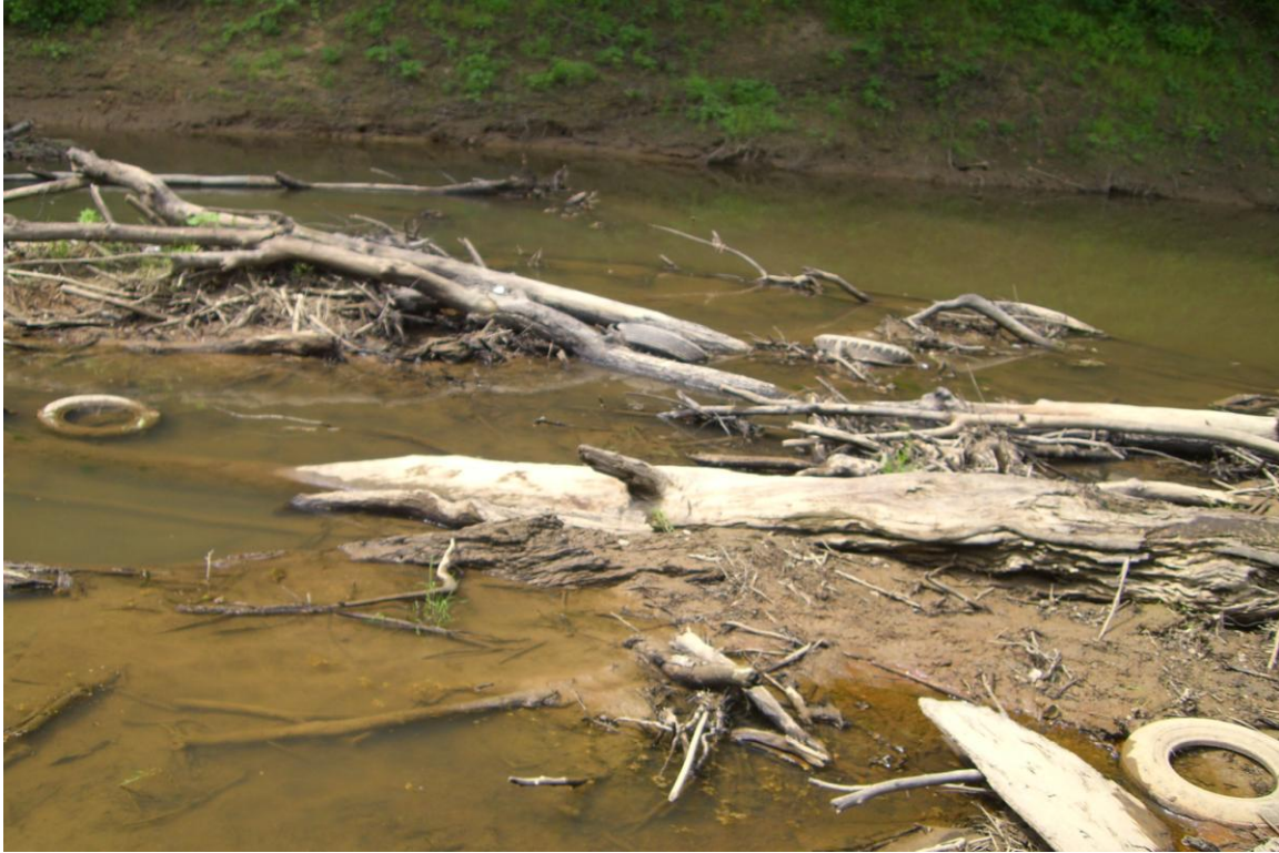
Figure 3. Photograph of the survey area for SCI 823-0.00/6.81 in the vicinity of the proposed bridge.
