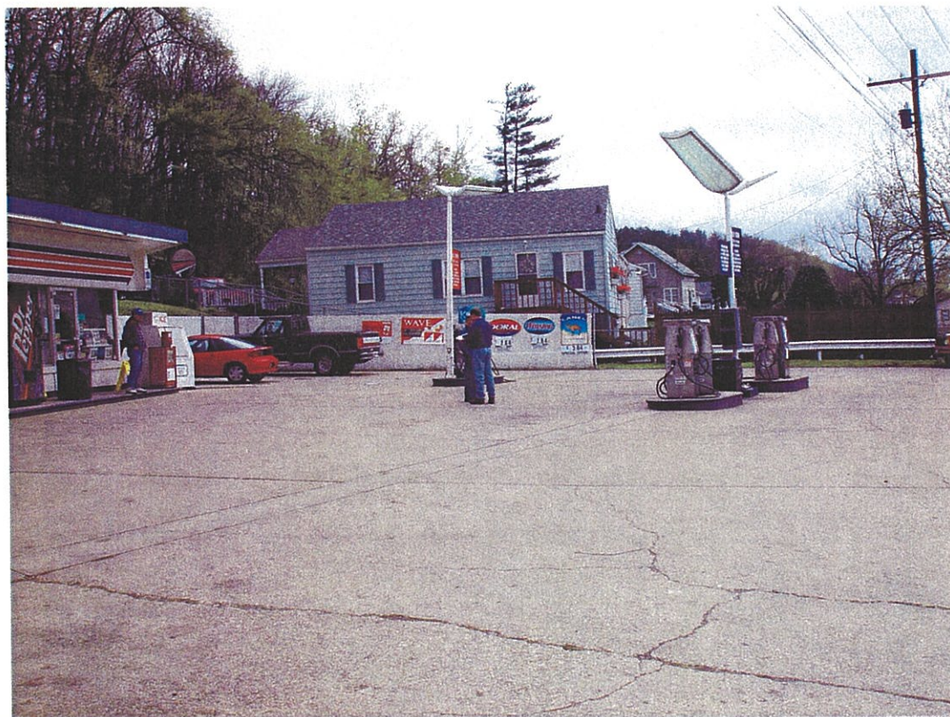
Photo 48. View looking east at the Buster's Bi-Lo property UST system and fuel island location.
