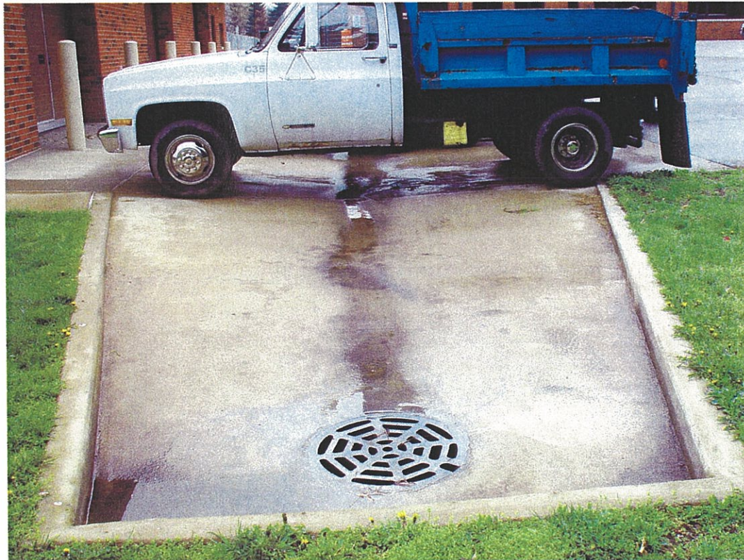
Photo 44. View of the Valley Middle School LUST property looking at the storm drain.
