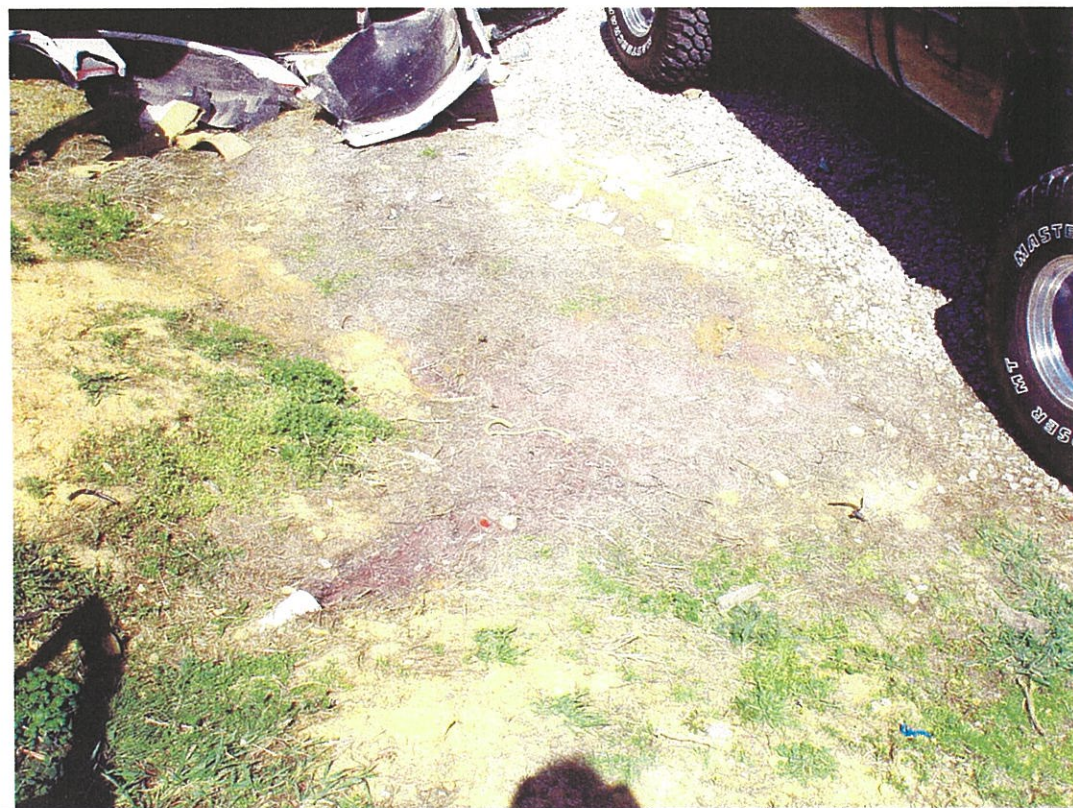
Photo 18. View looking at the area that the trench drains discharge onto the ground surface.
