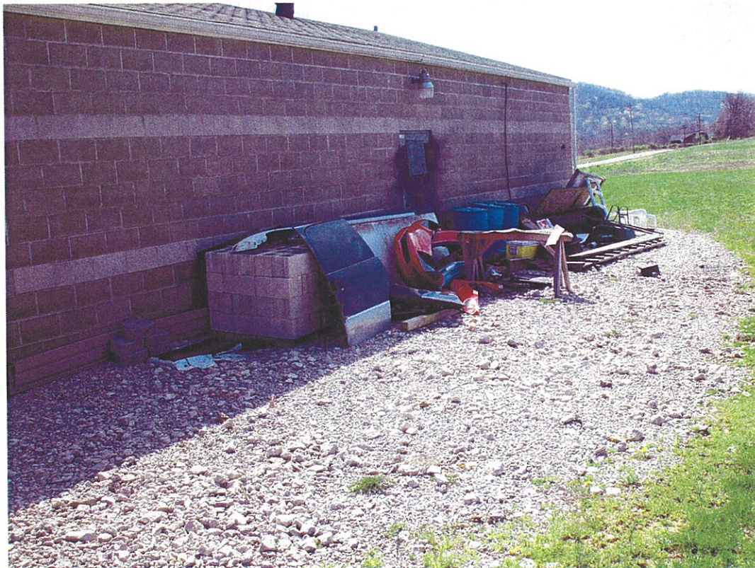
Photo 4. View looking at the rear of Kellers Collision building.
