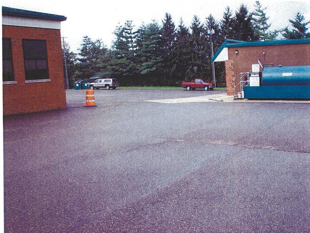
Photo 42. View of the Valley Middle School LUST property looking west along the northern portion of the property.
