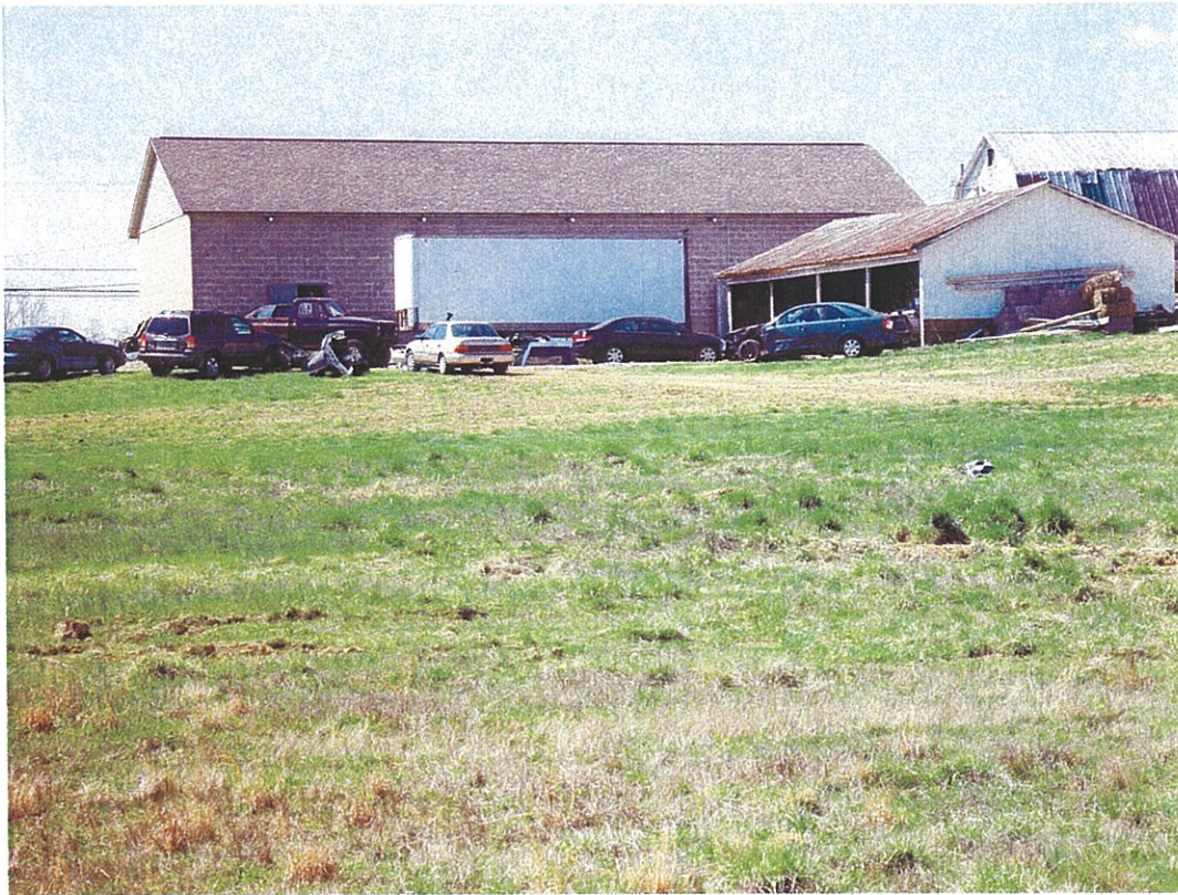
Photo 7. View looking at the rear of the auto repair garage located on Terry Turners property from the northern property boundary.
