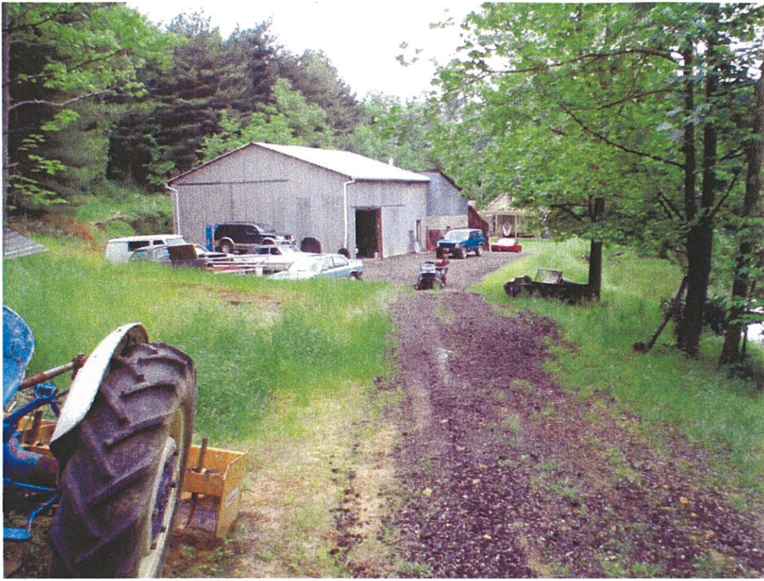
Photo 5. View of the maintenance facility, facing east.
