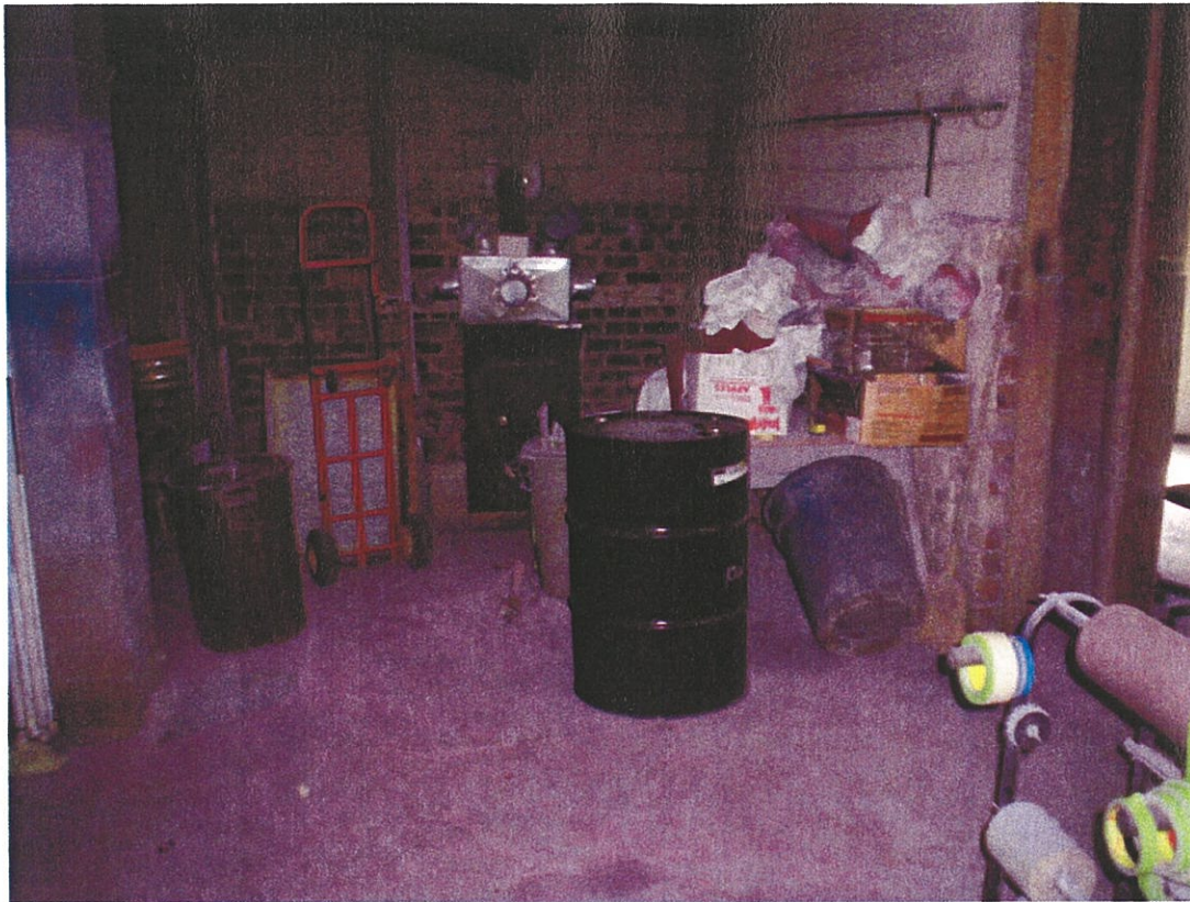
Photo 7. View of drum and debris.
