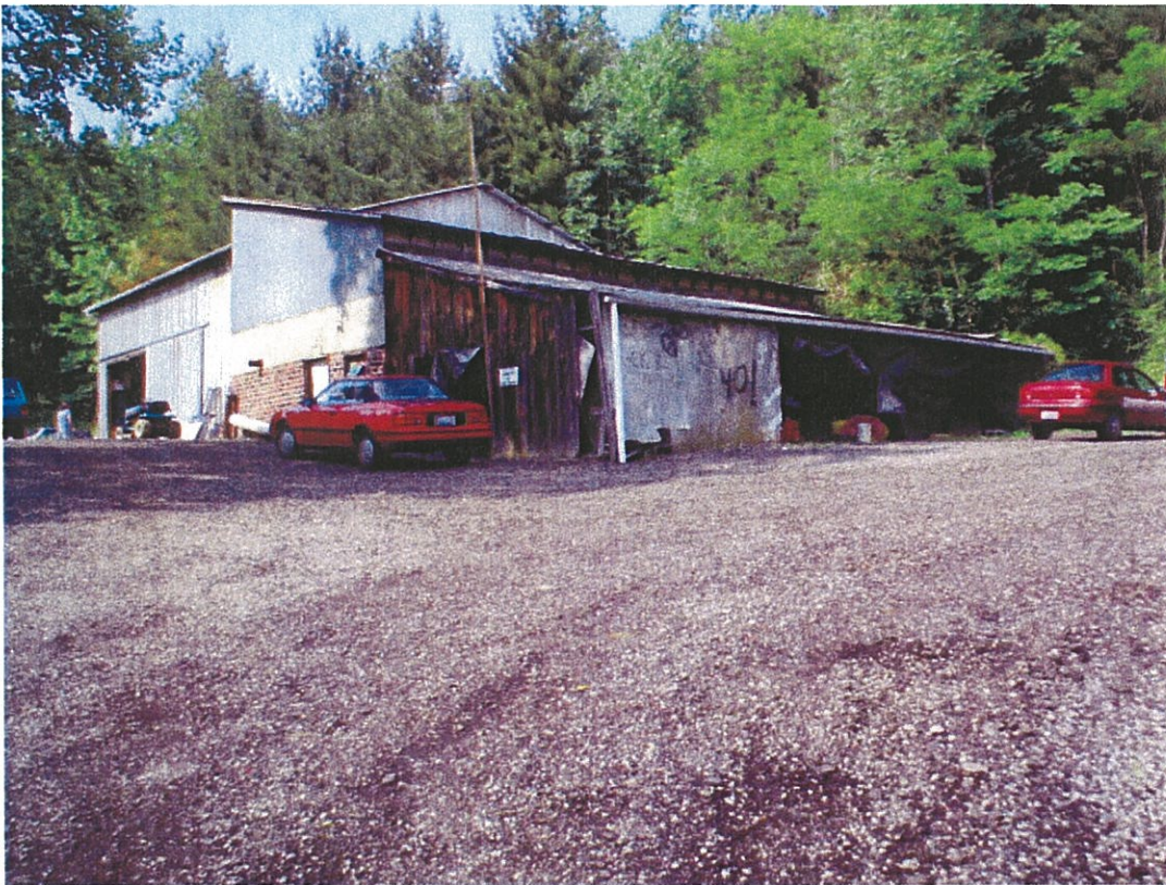
Photo 13. View of exterior of maintenance facility, facing north.
