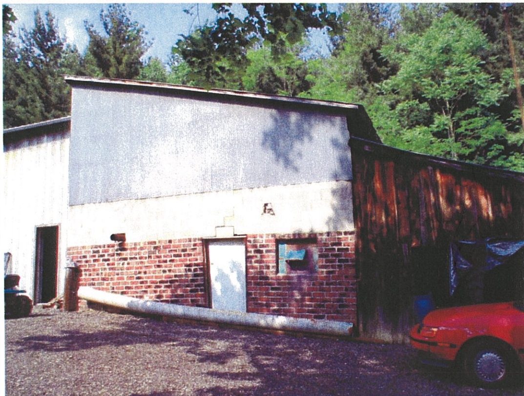
Photo 16. Exterior view of storage area, facing north.
