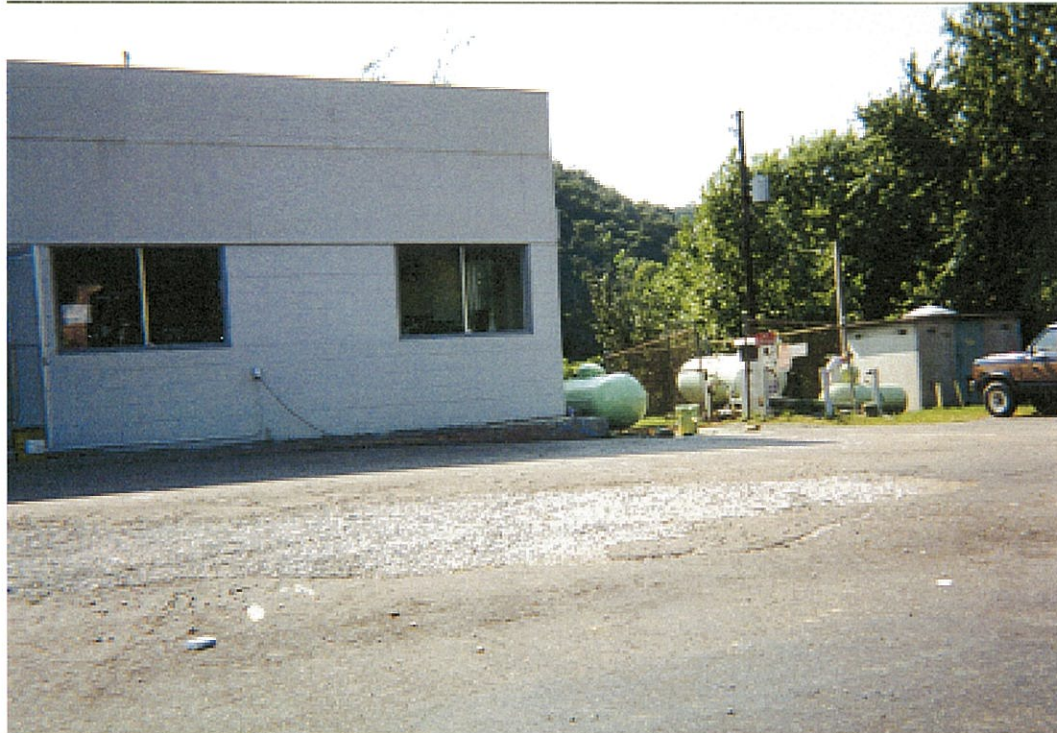
Photo 15. Arrick's Facility at Intersection of St. Rte. 139 & Co. Road 549, former gas station (tanks removed).
