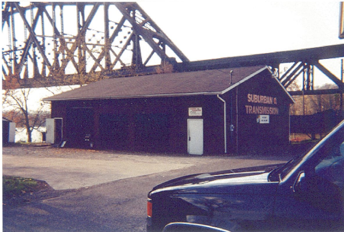
Photo 38. Suburban Transmission located between the Ohio River and U.S. 52 in southwest corner of corridor.
