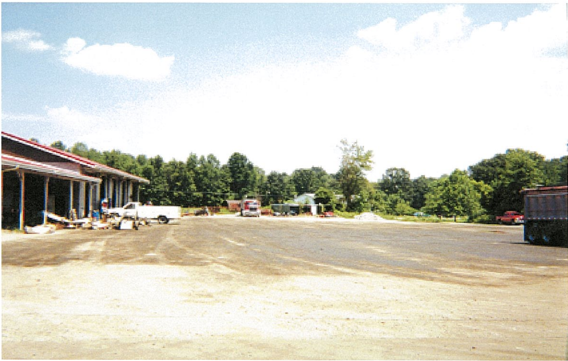
Photo 25. Oil stained lots at Conley Trucking.
