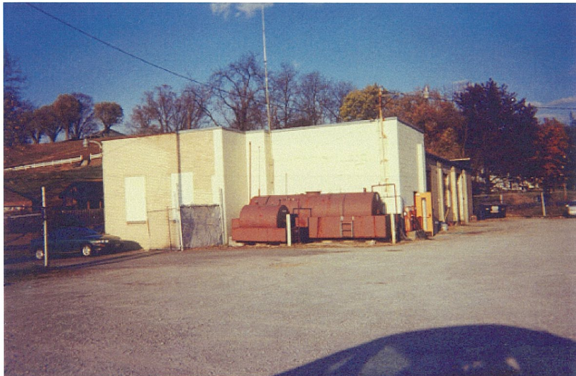
Photo 45. Fueling tank at the Wheelersburg Bus Garage.
