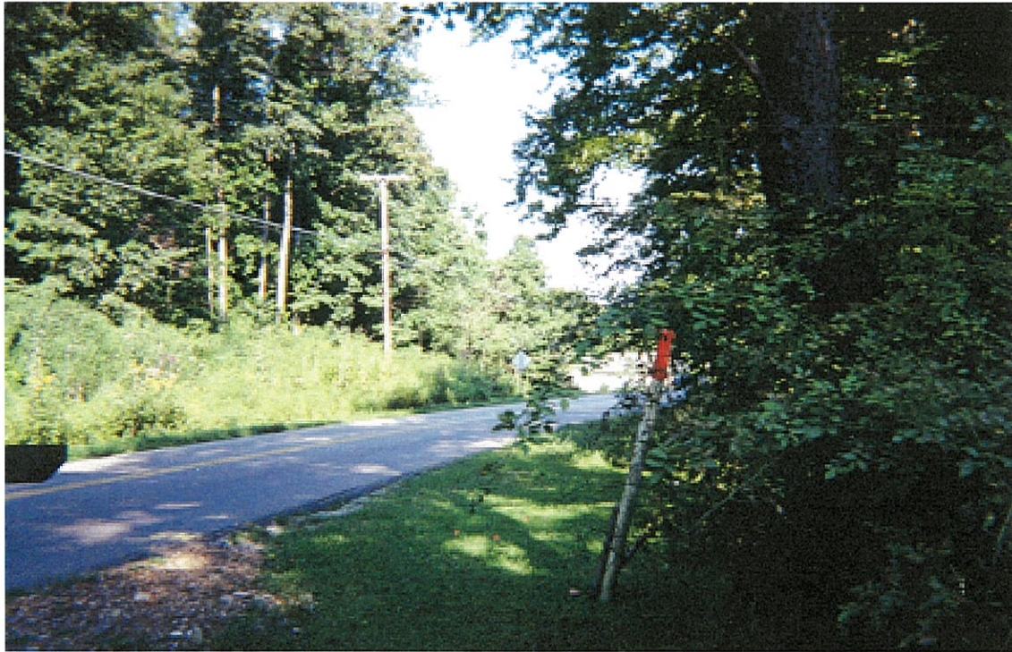
Photo 9. Gas pipeline and easement along Rte. 728 (facing west).
