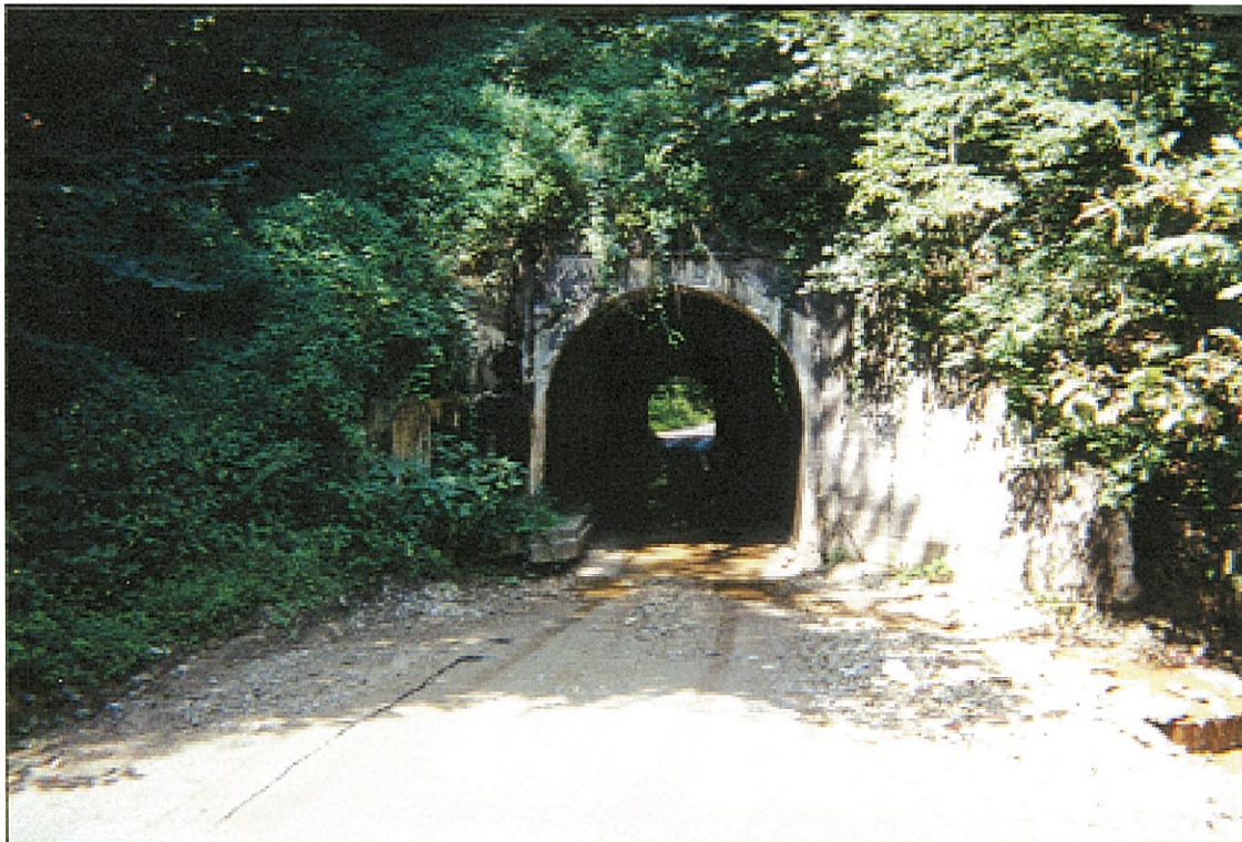
Photo 19. Tunnel/Bridge under railroad track along Blake Hollow Road, near St. Rte. 335.
