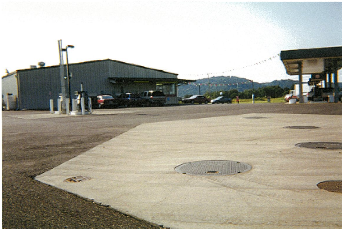
Photo 6. (Shell Oil) Retail Station site on St. Rte. 728 (facing SE) with monitoring wells.
