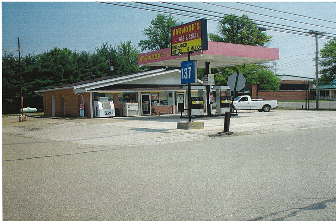
Photo 8. View looking northeast at Harwood's gas station from State Route 728, PID 240824000.
