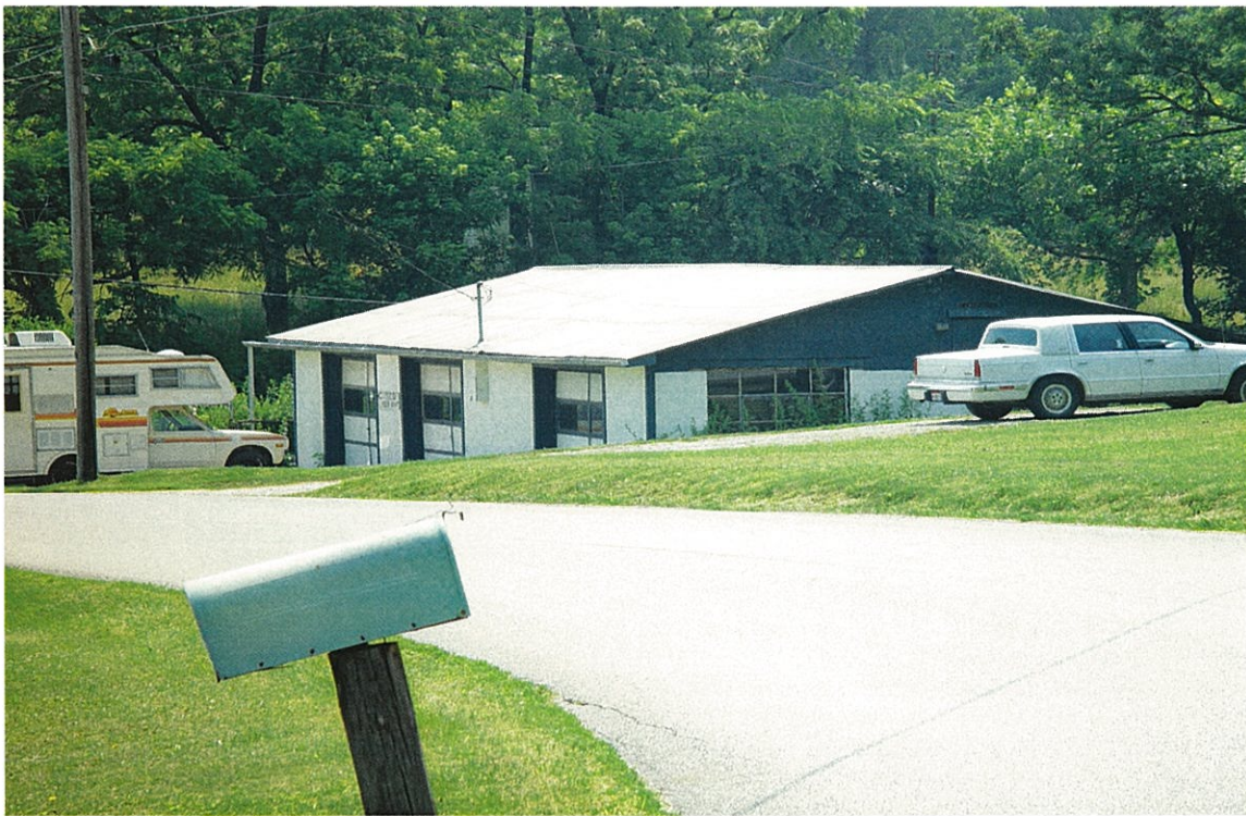
Photo 25. View of former service garage located at Slocum Ave and Dixon Mill Road, PID 160431000.
