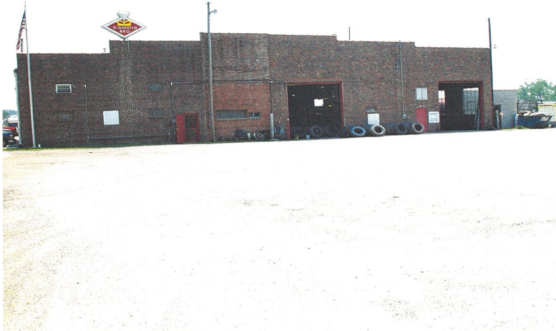
Photo 29. View looking south at the Diamond REO truck repair facility, PID 170666000.
