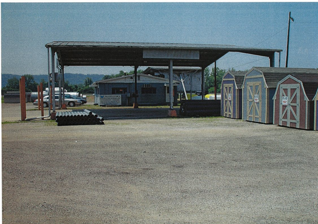
Photo 32. View looking Tri-State Culvert and Construction Supply facility, PID 170641001.
