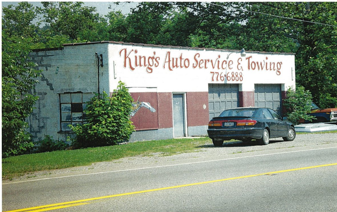
Photo 17. View of abandoned service facility located on State Route 140 (outside study area), PID 161165000.
