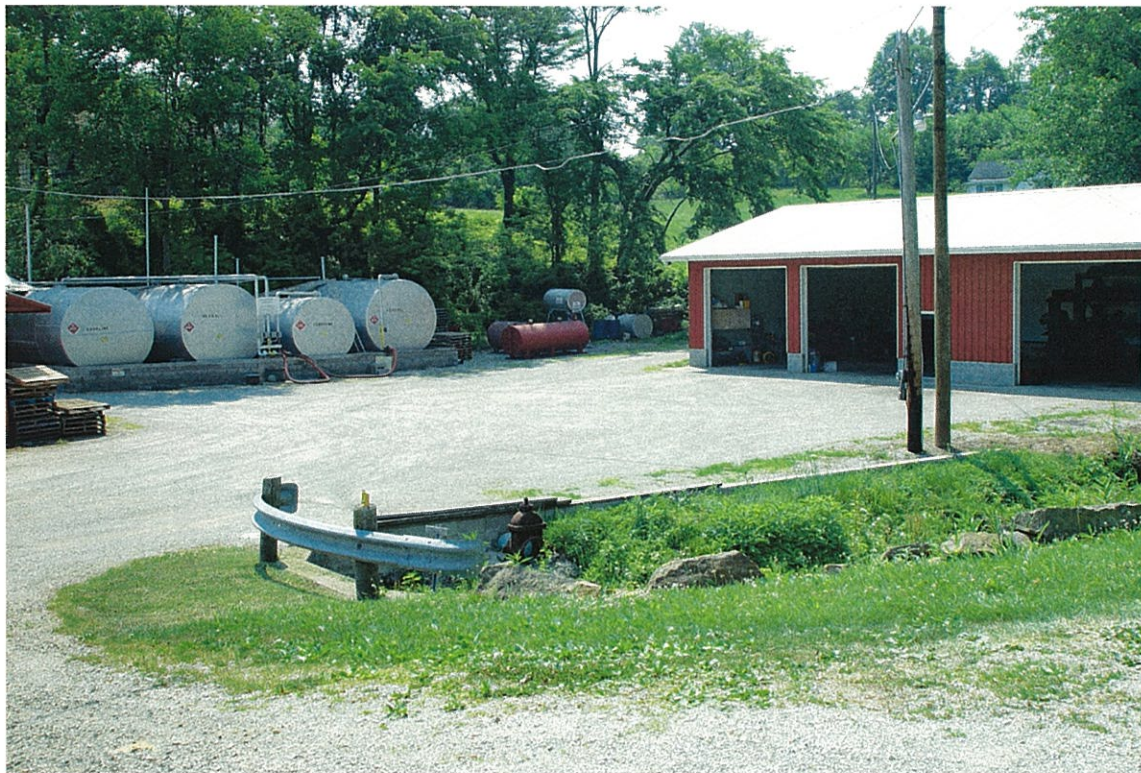
Photo 21. View of the ASTs behind Gerlach Farm and Feed facility, (Gampp's property) PID 160207000.
