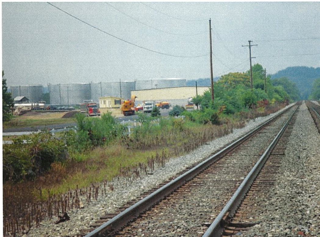
Photo 28. View looking northwest at the Kokosing Materials Inc. facility from the intersection of Center Street and the railroad tracks, PID 170733000 and 170735000.
