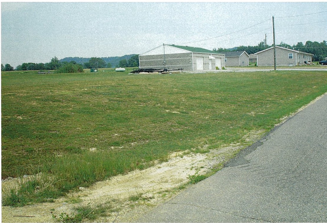
Photo 27. View of the Kellers Collision facility located at 133 Morris Lane, PID 080401012.
