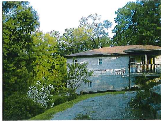
House used for receptor H2.
