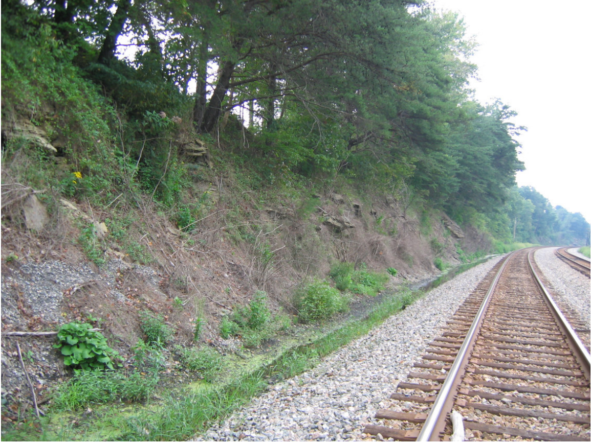
Photo 2. Bedrock Exposure: CSX Railroad cut.
