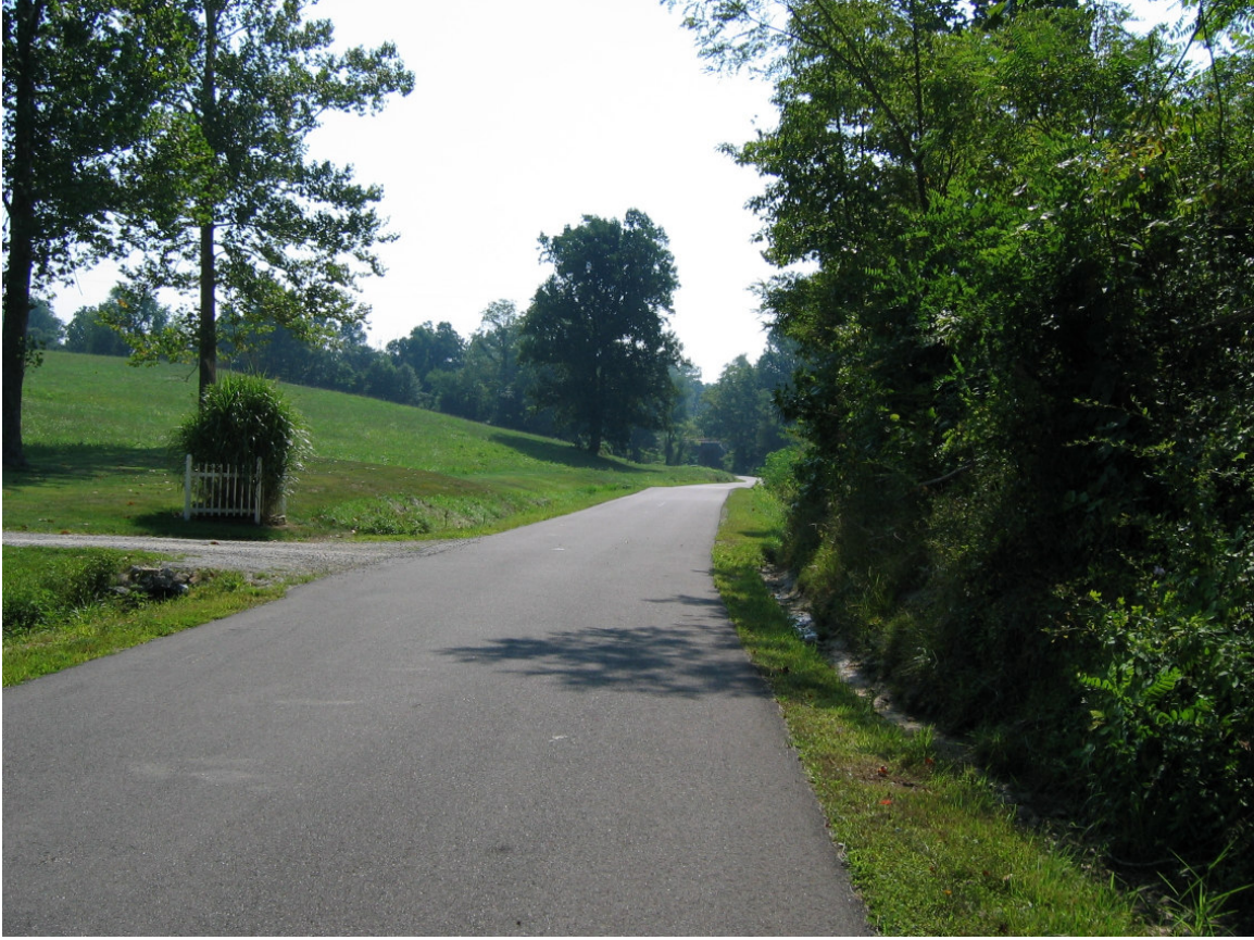
Photo 9. Pavement: Shumway Hollow Road.
