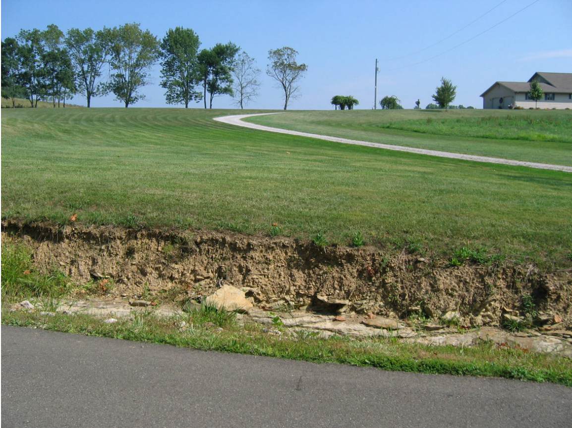
Photo 1. Bedrock Exposure: Shumway Hollow Road Ditch
