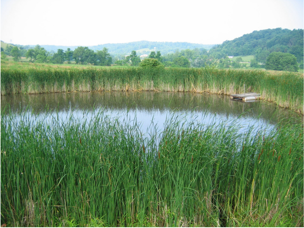
Photo 7. Excavated embankment pond near Sta. 531+00
