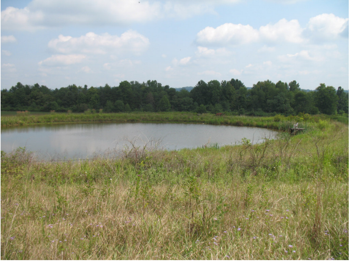
Photo 5. Spring-fed excavated embankment pond near Sta. 410+50.
