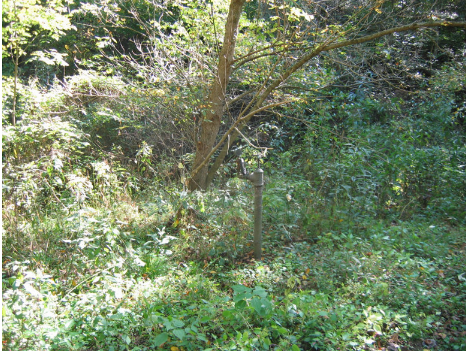
Photo 3. Previously unknown gas well 760 feet left of station 659+00.
