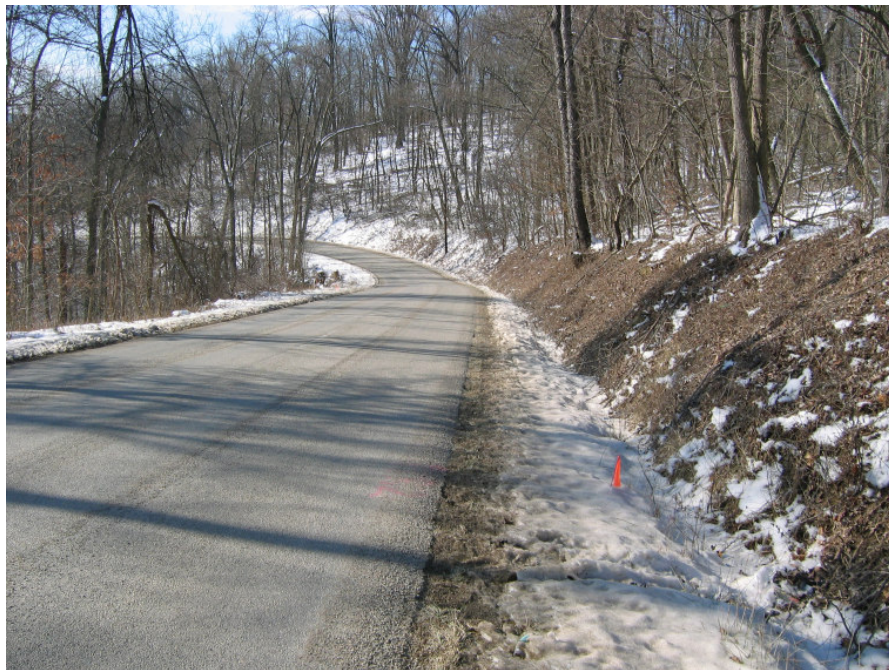
Photo 12. Flatwoods-Fallen Timbers Road
