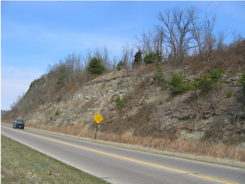
Photo 11. Rock cut at station 44+00.
