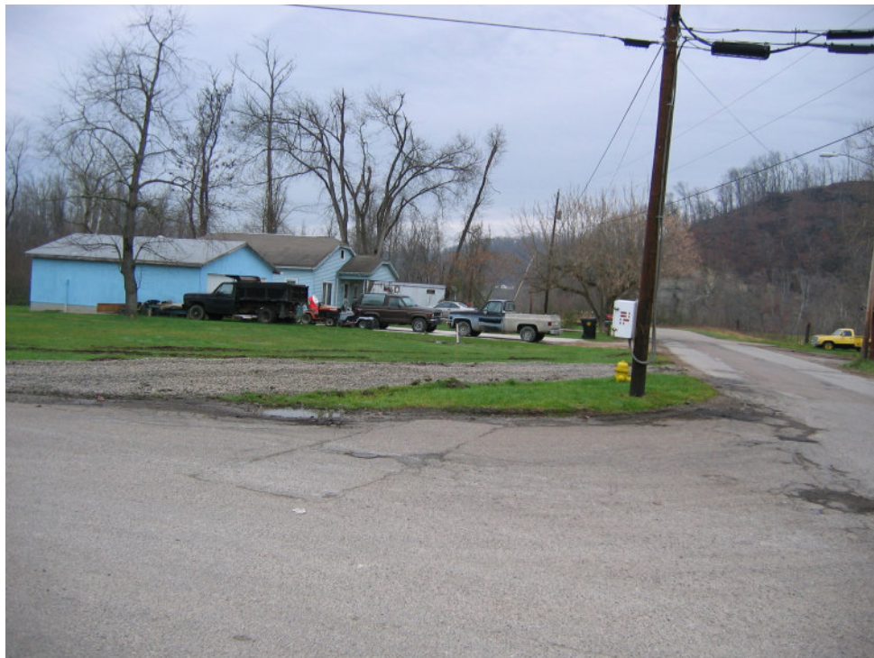
Photo 2. Pershing Avenue. and Slocum Avenue asphalt pavement
