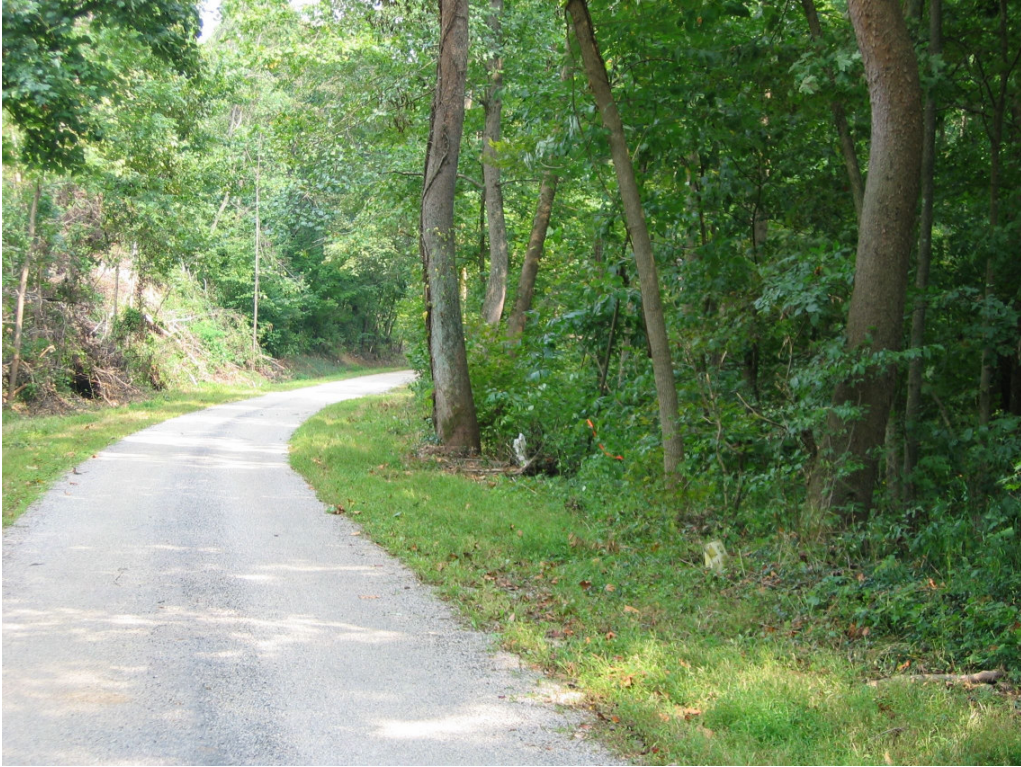
Photo 5. Blake Hollow Road chip seal pavement.
