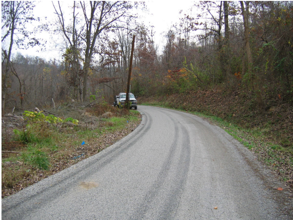
Photo 4. Stout Hollow Road chip seal pavement.
