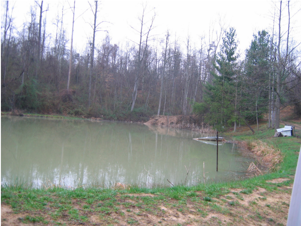
Photo 7. Excavated embankment pond at Station 73+50.
