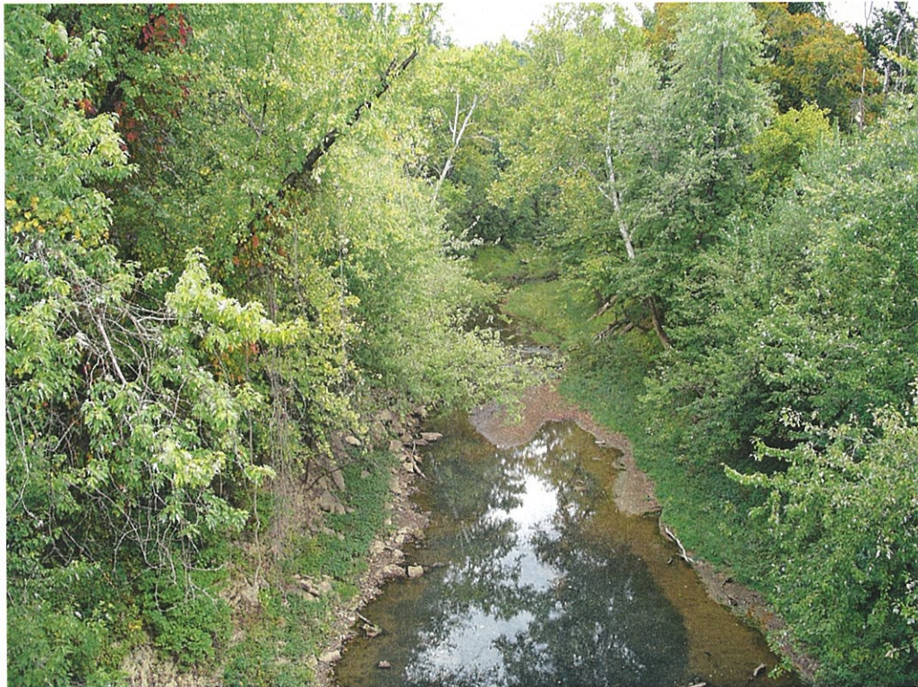
Upstream of Existing Slocum Road Bridge
